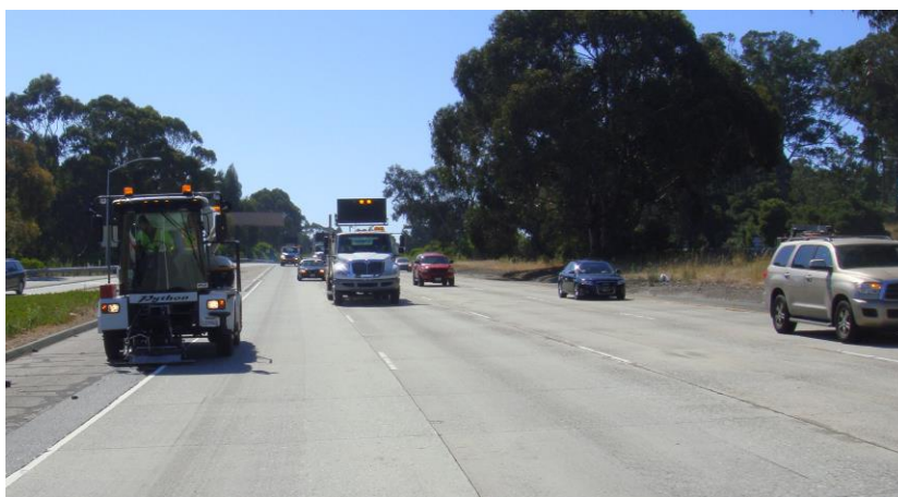
Figure 4. Caltrans Moving Closure Patching Operation
