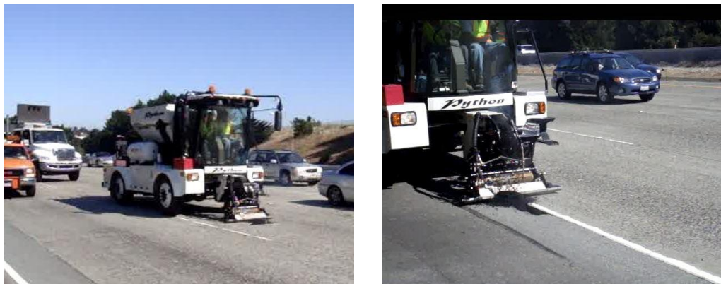
Figure 3. Python PHP Asphalt Patching Operation – Moving Closure on Interstate (I) 280
