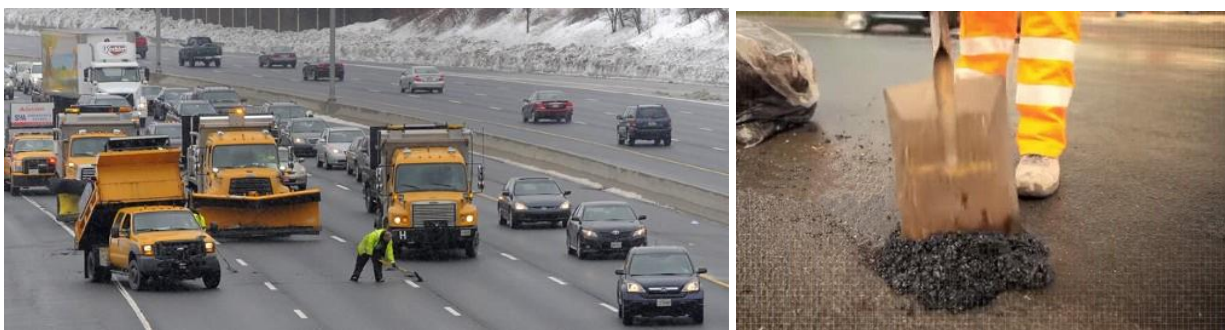
Figure 1. Manual Pothole Patching on Mainline Highway
