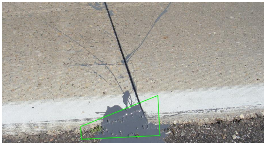
Figure 32. Caltrans Urethane and Gravel Spall Patch – Interstate 8
