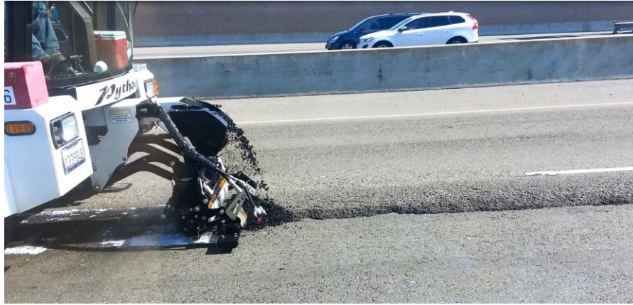
Figure 21. Linear Pavement Gap Patching
