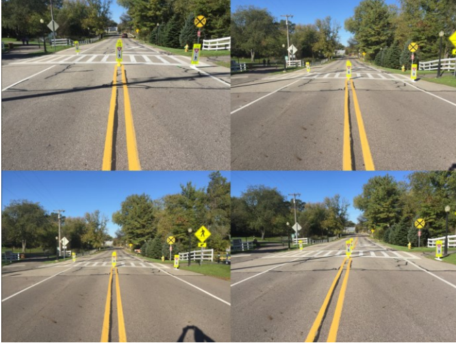
Figure 5.1 Photographs of different Gateway widths: (Top left) 12ft, (top right) 14ft, (bottom left) 16ft, and (bottom right) 18ft.
