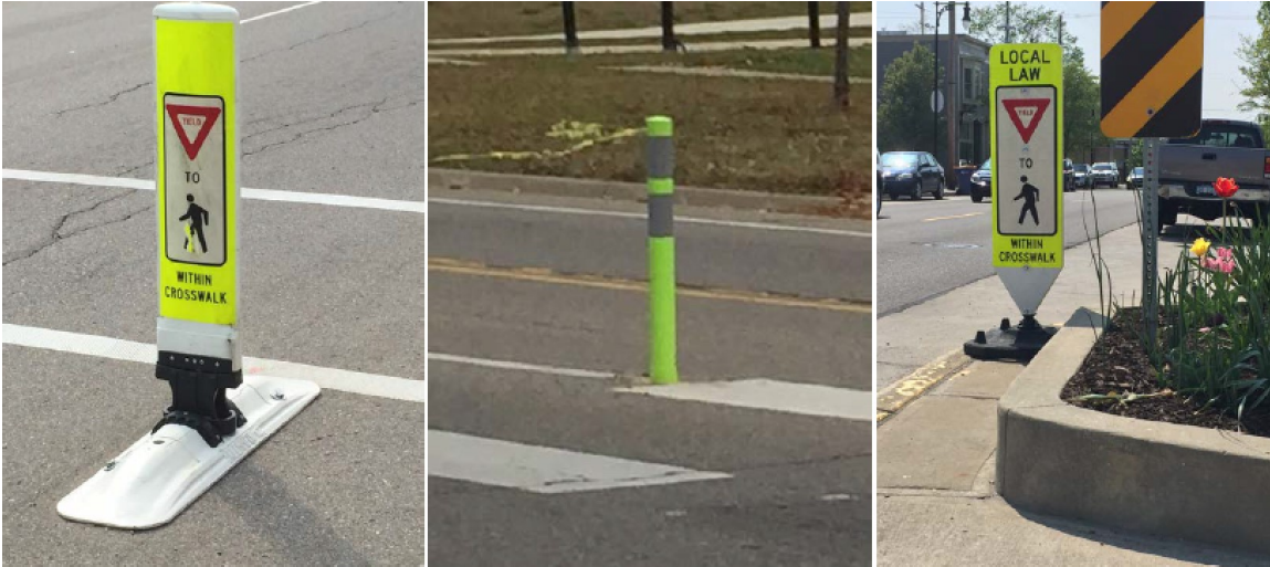
Figure 3.1. Figure 3.1a (above left) shows an R1-6 sign installed on a removable curb base. Figure 3.1b (middle) shows a flexible delineator installation. Figure 3.1c (above right) shows an R1-6 sign mounted on a flush mounted base.
