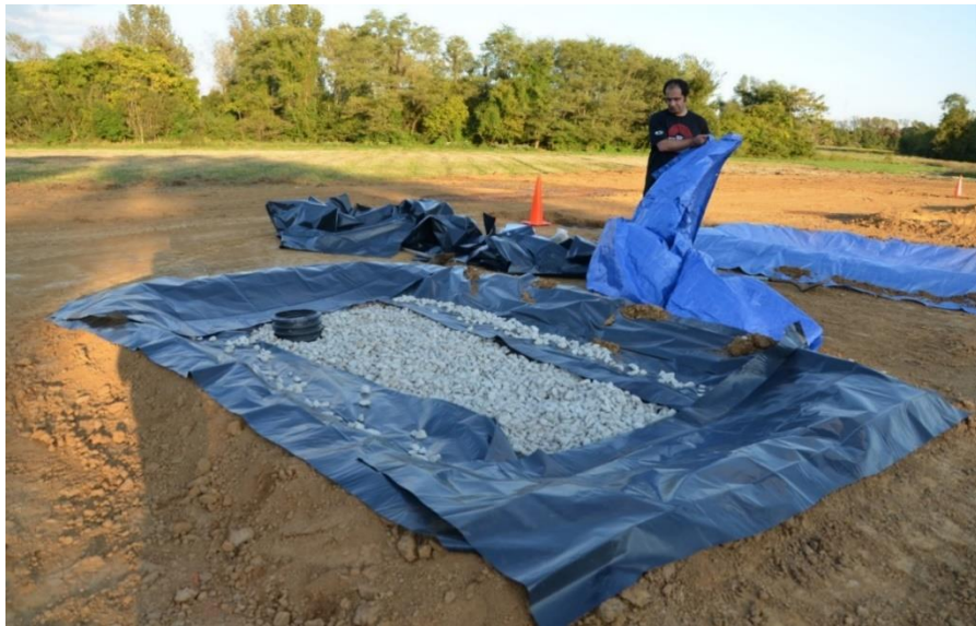
Figure 42. Heavy-duty plastic to cover perimeter berm and tarp to cover the entire test cell.
