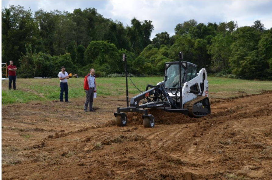
Figure 39. Clearing and leveling off the ground.
