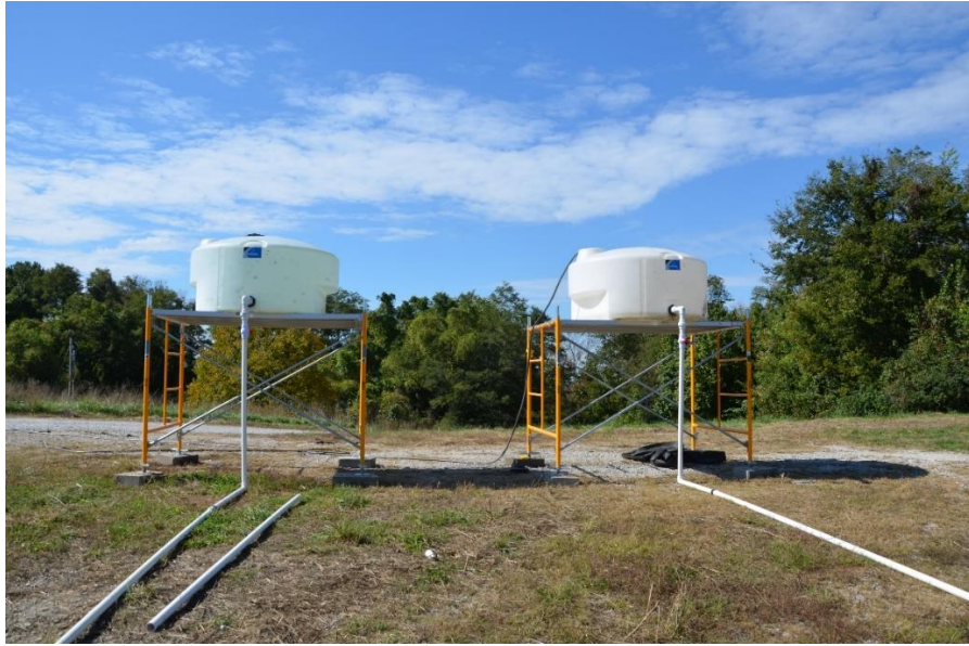
Figure 38. Two 300-gal water tanks on scaffold.
