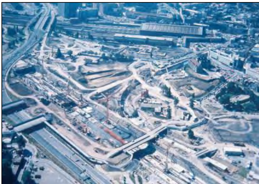
Figure 12. Aerial Photograph of the Euralille Construction Project
