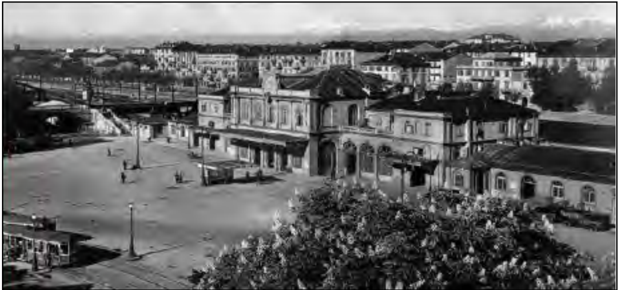
Figure 53. Original Torino Porta Susa Station (1800s)
