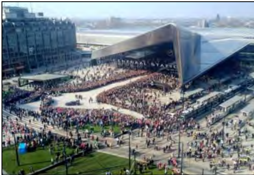
Figure 38. The Station Façade to the South, with its Integrated Large Plaza, at its Grand Opening in 2014
