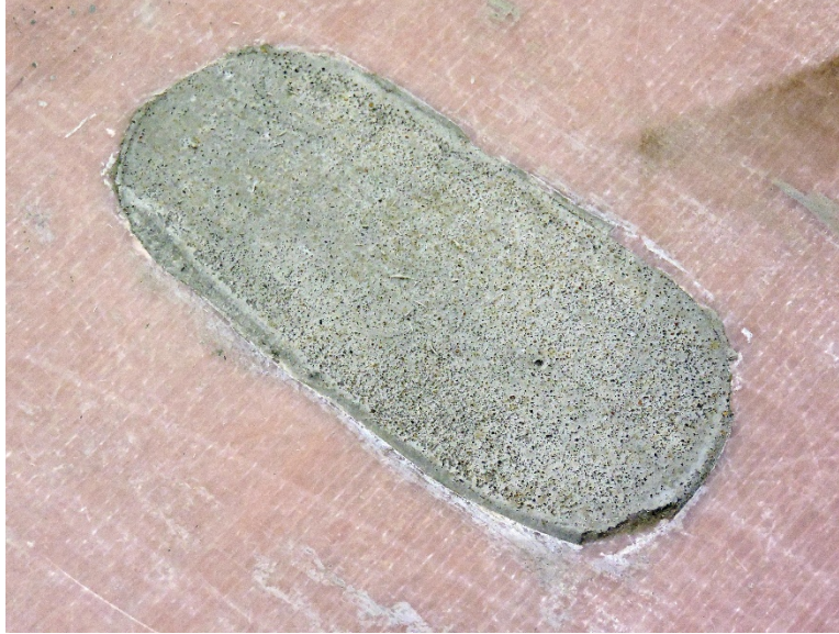
Figure 8.2: Headed Shear Stud Pocket After Grouting
