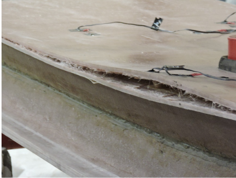
Figure 6.2: Local Buckling of Compression Flange, Specimen FP-1
