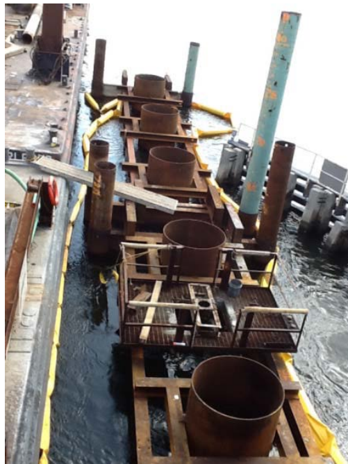
Figure 1.4 Construction of drilled shafts with casing
