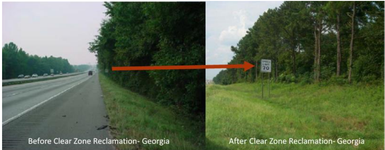
Figure 6.1 Sign visibility and roadside clear zone before and after clear zone reclamation in Georgia
