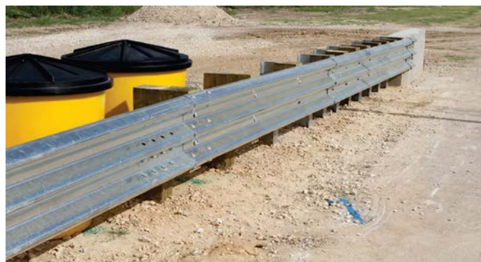
Figure 1.9. Test No. 467114-7 Installation Setup.
