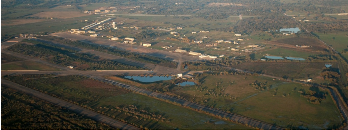
(a) Aerial View
