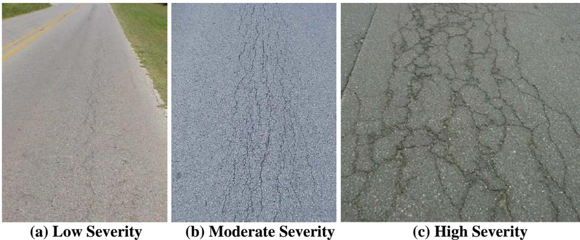
**Figure B-2. Alligator Cracking.**
