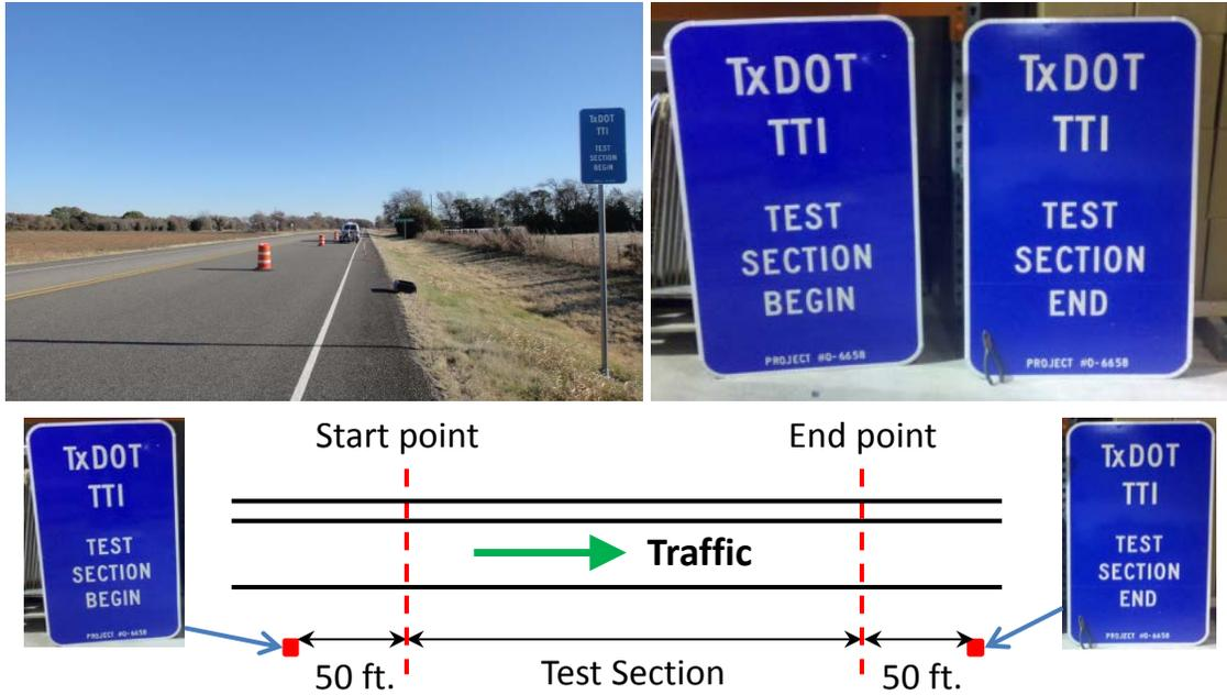
**Figure 5. Installation of Road Signs at Test Section.**
