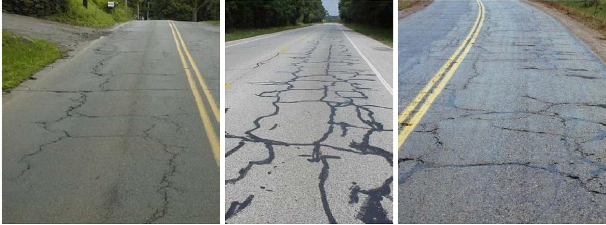
**Figure B-4. Block Cracking.**
