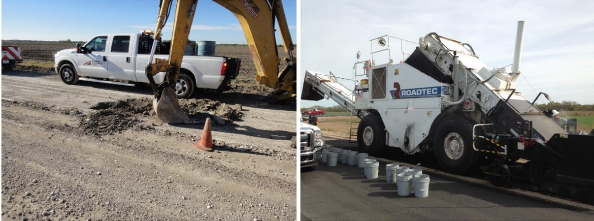
**Figure 13. Sampling Base and HMA Materials during Construction.**
