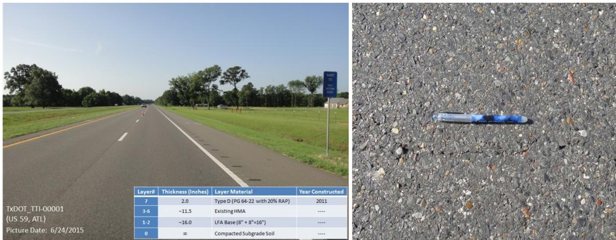
**Figure 23. Google Picture and Surface Cracking on US 59 Section (Atlanta District).**
