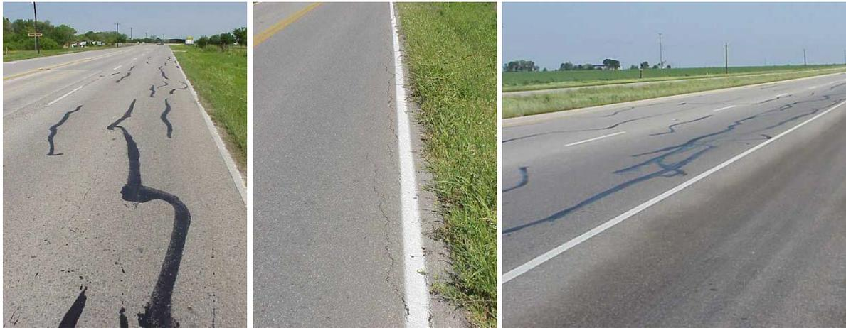
Figure B-6. Longitudinal Cracking.
