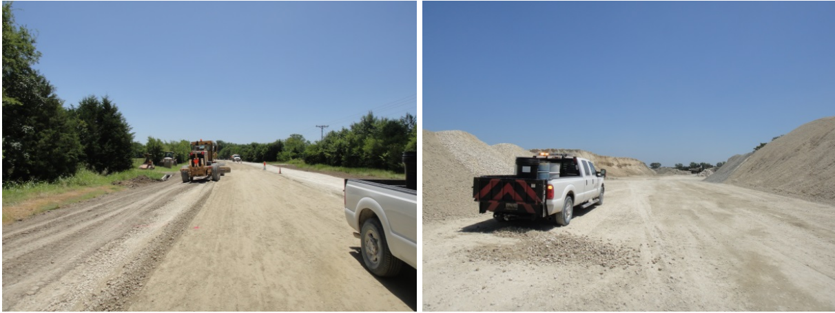
Figure 6. Sources to Collect Base Material: (a) Construction Site and (b) Quarry.
