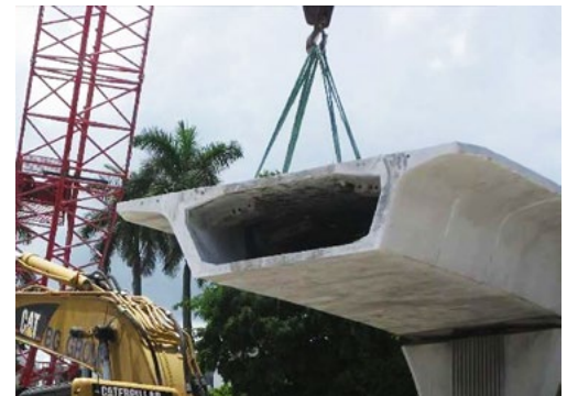
Segments from this decommissioned ramp were used to evaluate non-destructive testing methods.
