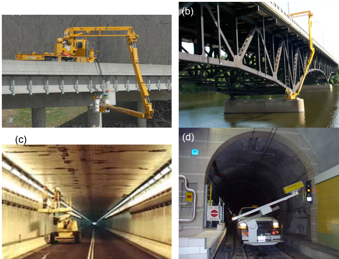
Fig. 2. Examples of bridge, railway, and tunnel inspection (a) Concrete bridge inspection (MN-DOT); (b) Steel bridge inspection (MO-DOT); (c) Tunnel inspection (FHWA); (d) Railway tunnel inspection using GPR
