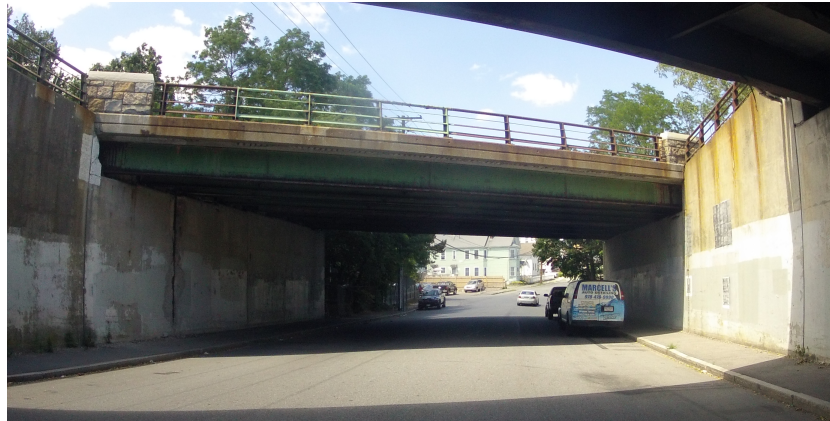
Fig. 75. Bridge site # 1, L-15-074 Lowell Connector over Lincoln St.
