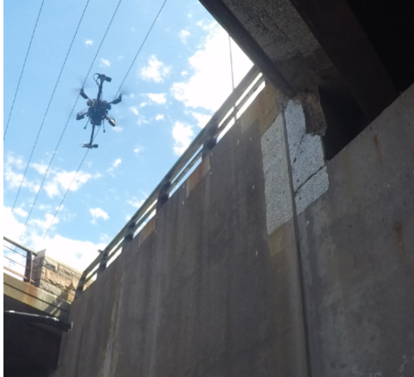
Fig. 85. UAV inspection being performed at monitoring area 1-5, Test date June 23, 2016.
