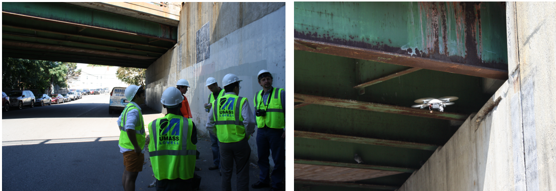
Fig. 102. Field validation of the CivilEye+Radar system at Lincoln St. Bridge, Lowell, MA
