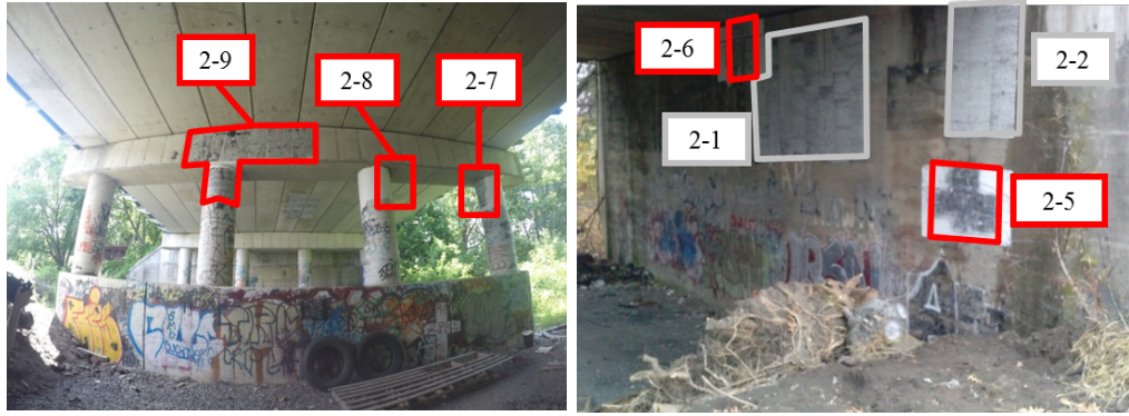
Fig. 96. Inspection areas at bridge site #2 – Plain St. over CSX Railway
