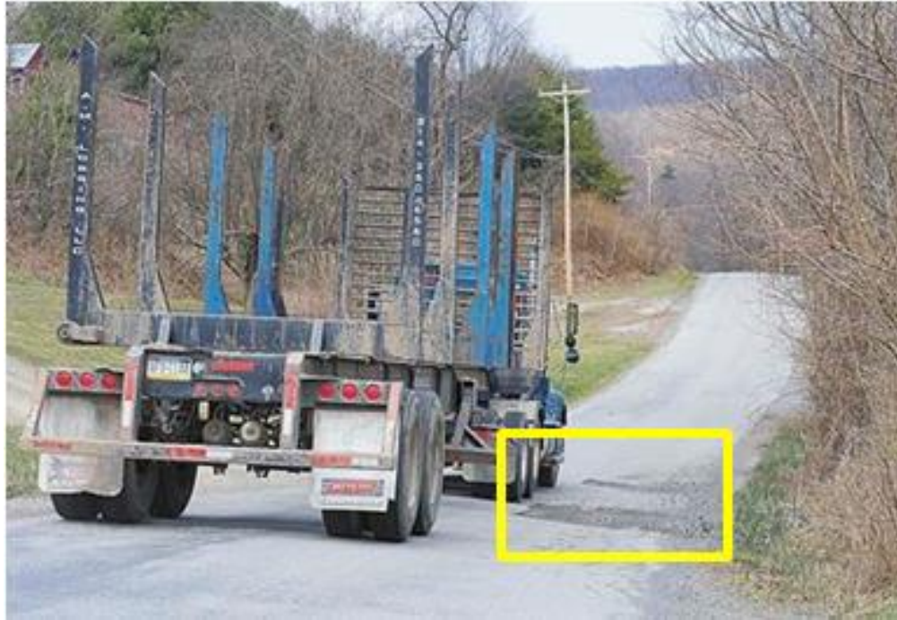
Figure 2: Roadway damage due to frost – thaw conditions and uncontrolled use
