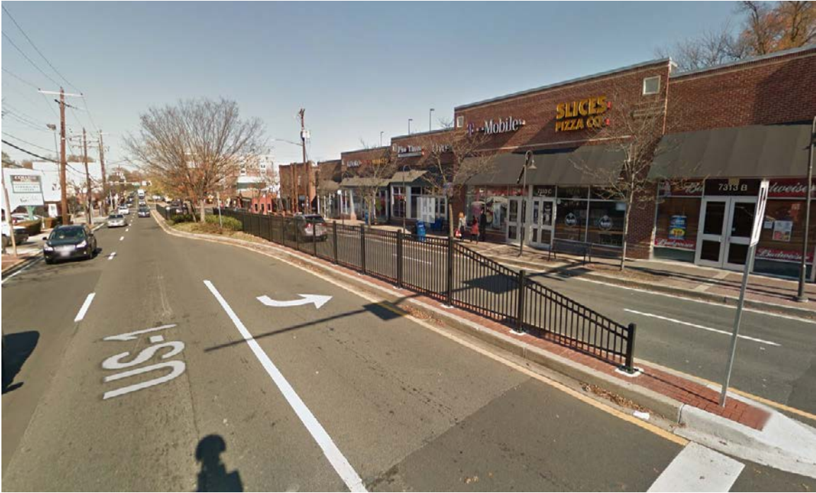
Figure 22: Fencing College Park- US 1
