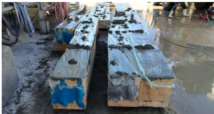
Figure 3.1-3– RC Beam concrete casting
