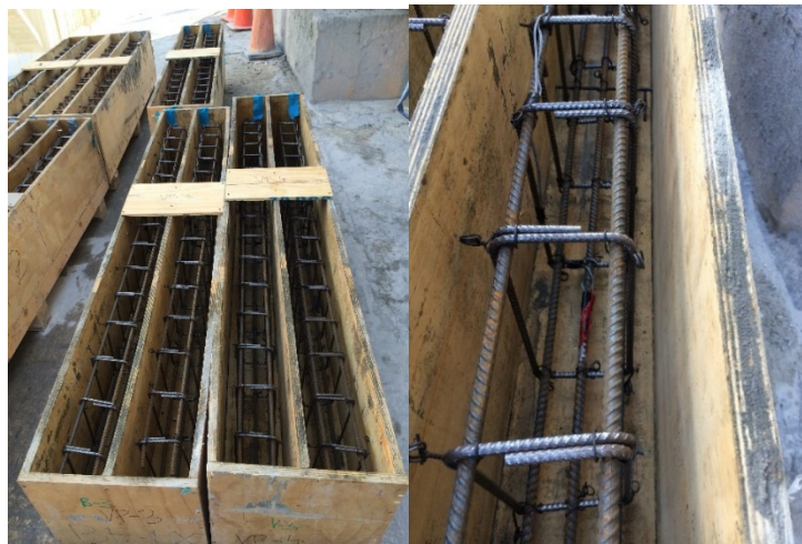
Figure 3.1-2– RC beam preparation
