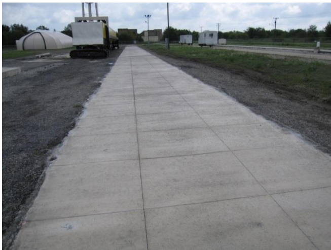
Figure 3.1 Constructed full-scale thin FRC overlay, view of section 1.
