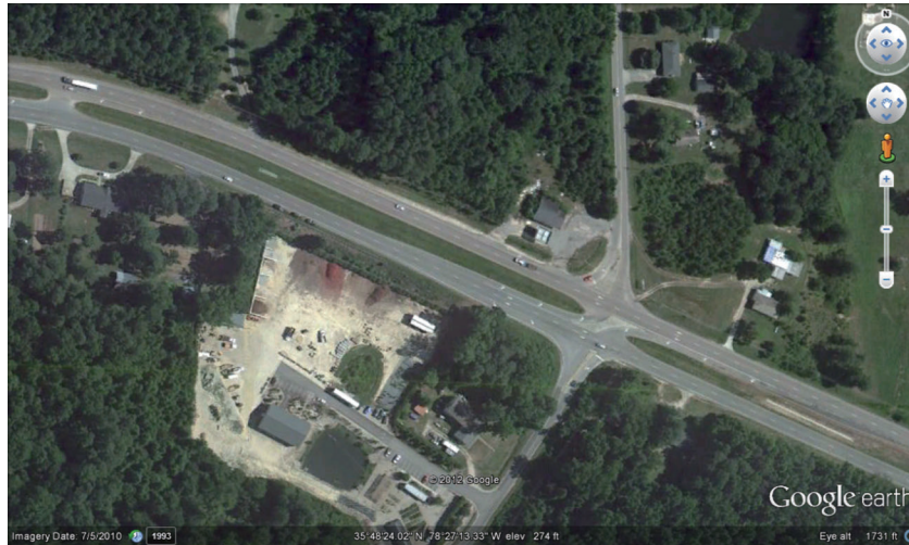
Figure 6.5 J-turn intersection at US 64 & Mark's Creek Road in North Carolina (28).
