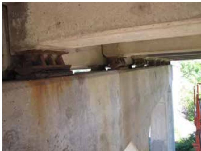
Figure 2.3: Support Rockers at Pier 4, Left Side, Span 5 of Bridge No. 54-104-317.27
