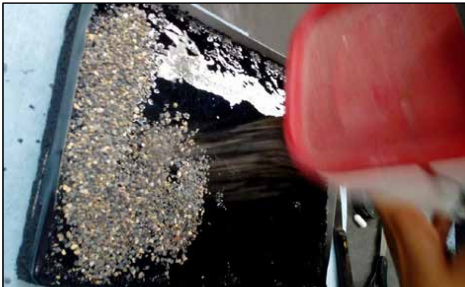
Figure 3.16: Aggregate Being Spread Over the Epoxy-Covered Slab
