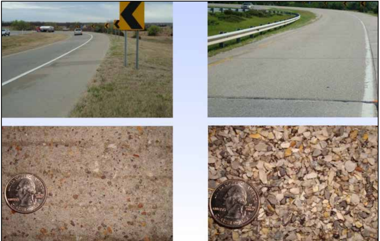
Figure 2.19: Before and After HFST on K-96/US-54 Ramp in Wichita (Concrete Pavement)
