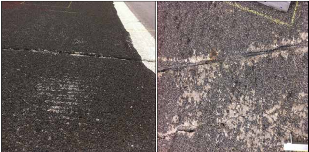
Figure 2.21: De-Bonding of High Friction Surface Aggregates
