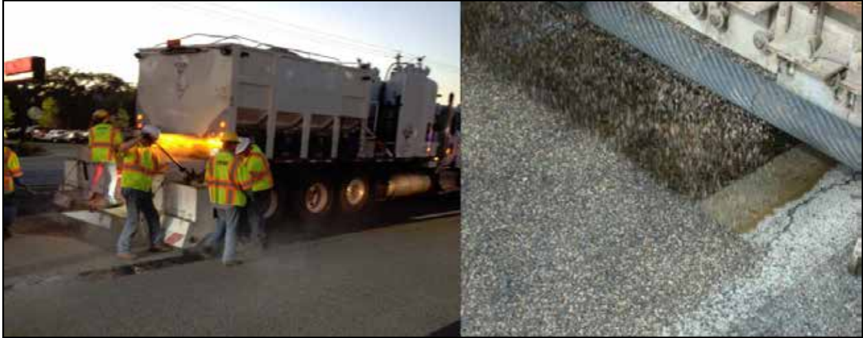
Figure 2.11: HFST Fully Automated Application
