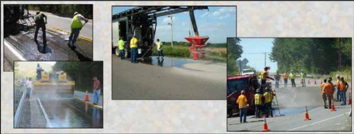
Figure 2.10: HFST Semi-Automated Application Source: FDOT (2015)
