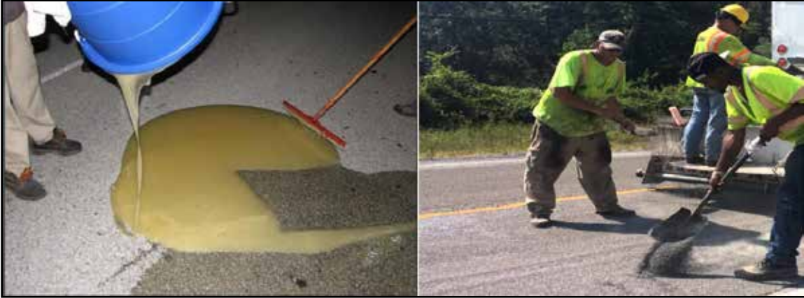
Figure 2.9: HFST Manual Application Source: FDOT (2015)
