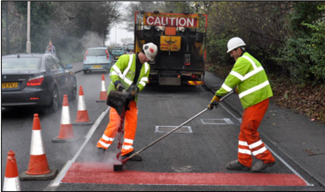
Figure 2.1: Hot-Applied HFST Source: Jointline Group Limited (2014)
