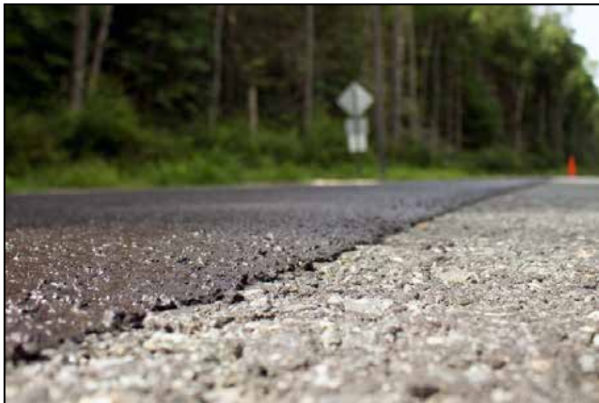
Figure 2.14: Typical Microsurfacing Treatment
