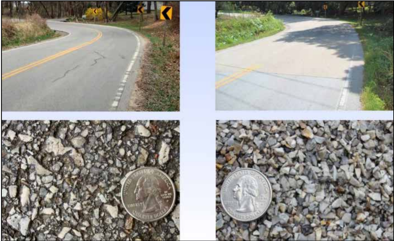
Figure 2.17: Before and After HFST on K-5 in Leavenworth County (Asphalt Pavement)
