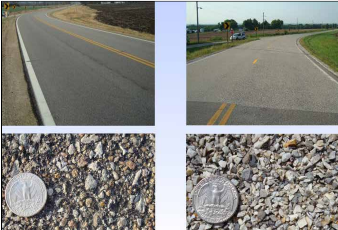
Figure 2.16: Before and After HFST on K-99 in Wabaunsee County (Asphalt Pavement)
