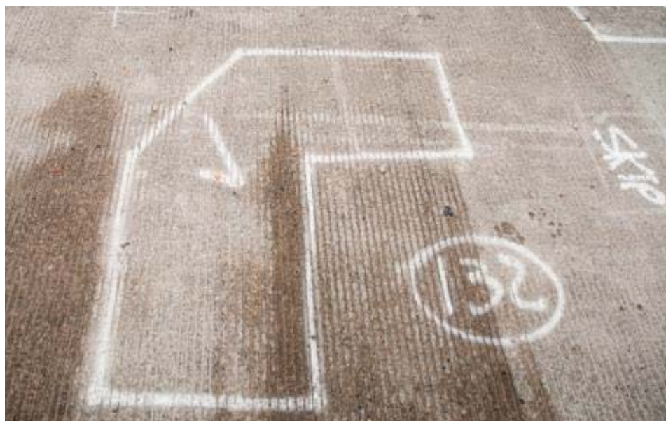
Figure 43: Sounding estimate of the I-55 bridge deck delamination 132.
