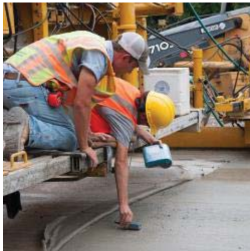
Figure 75: Fresh tie bar location identification with low-power rebar meter. Fresh concrete was removed to confirm tie bar measurements.
