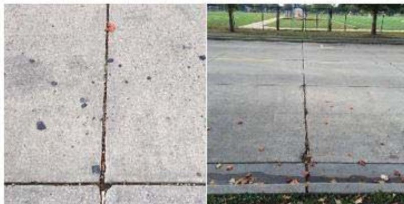
Figure 97: Stadium Drive with unsealed joints.
