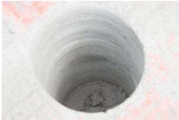
Figure 74: Visual dowel bar depth at an existing cored location.
