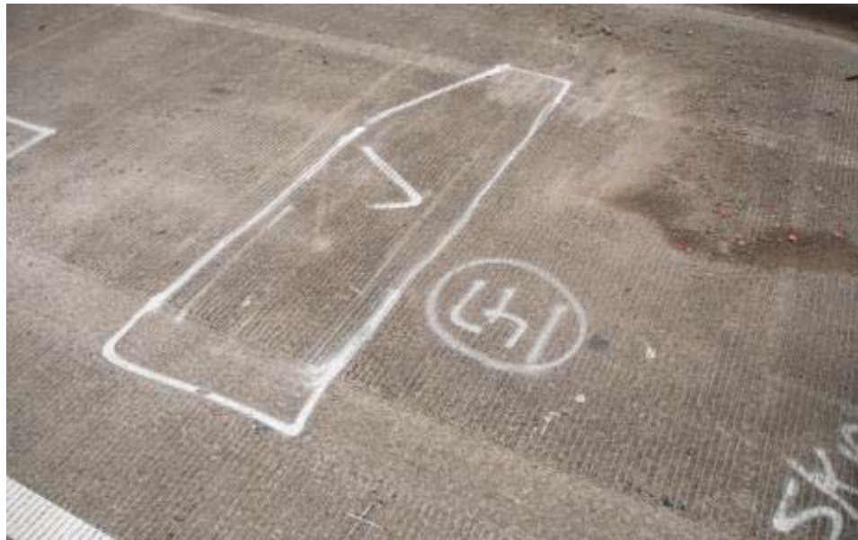
Figure 44: Sounding estimate of the I-55 bridge deck delamination 147.
