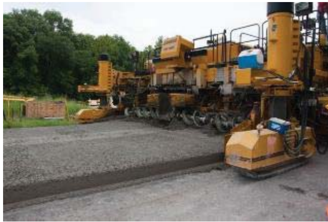
Figure 73: Two-lane slipform paver.
