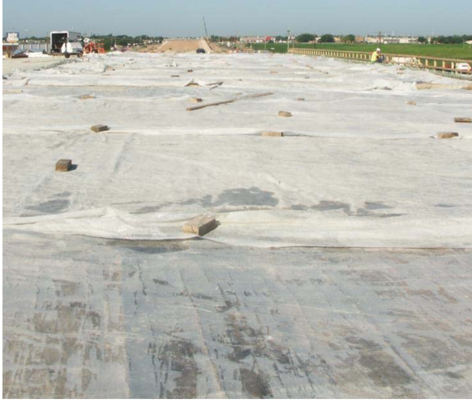
Figure 7.36: Curing method for Lubbock bridge deck.
