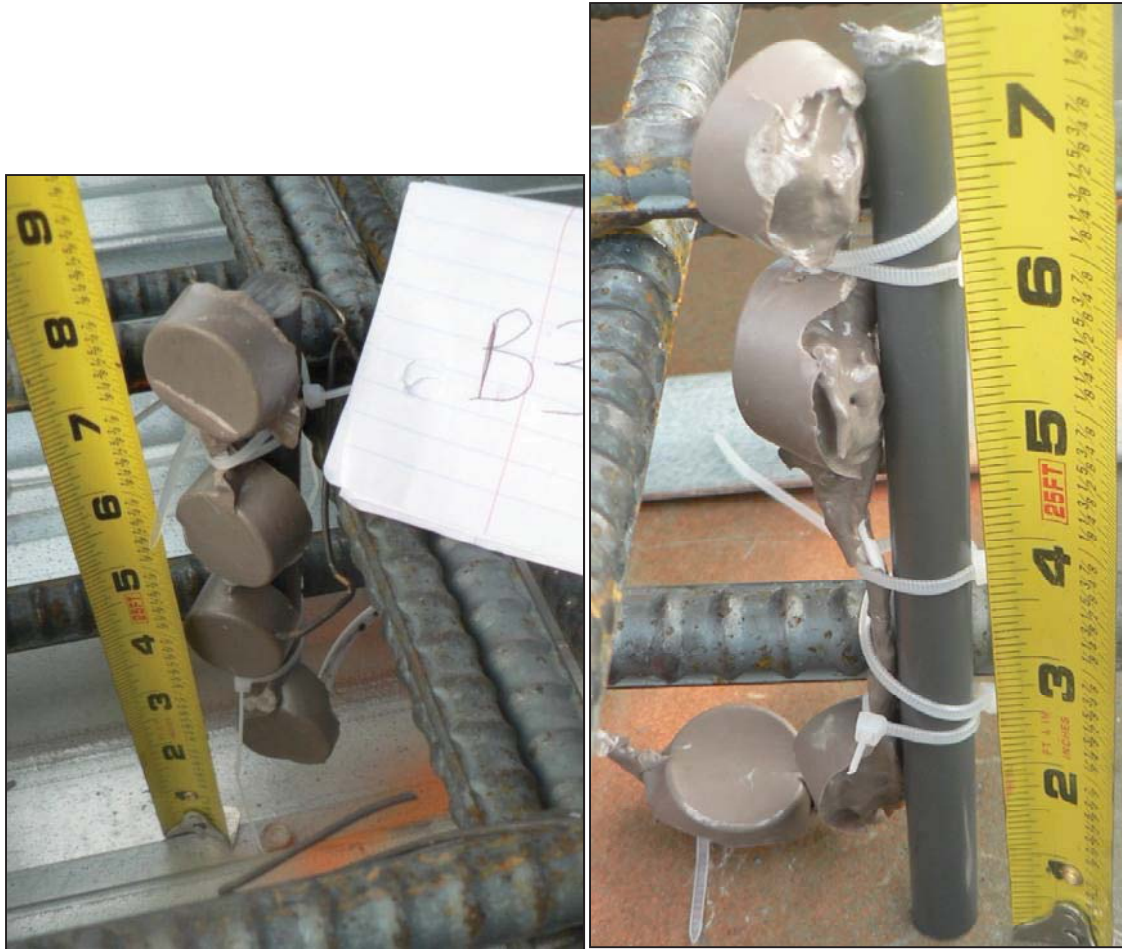
Figure 7.5: iButton strings for San Antonio bridge deck.
