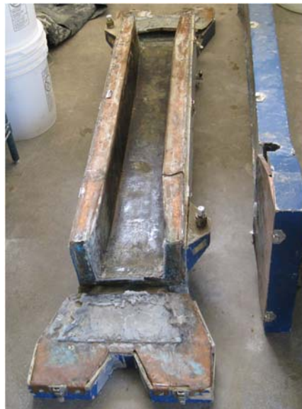
Figure C.3: Deterioration of existing formwork.
