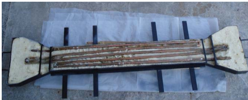
Figure C.10: Bottom formwork before application of flashing.
