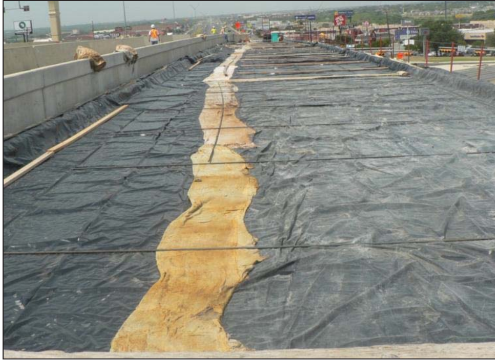
Figure 7.6: Curing method for San Antonio bridge deck.
