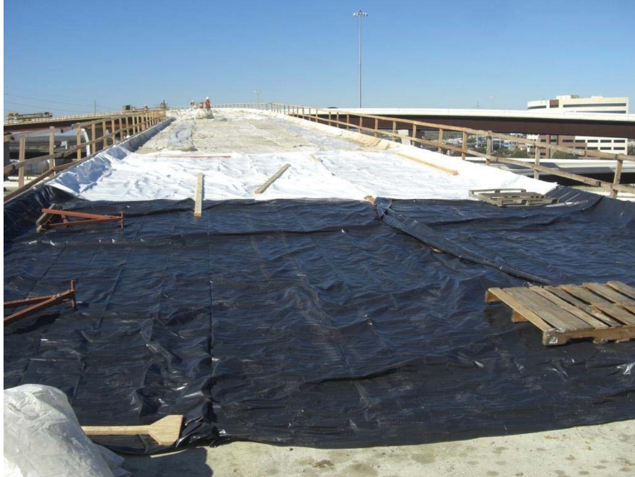
Figure 7.49: Bridge deck during removal of curing
