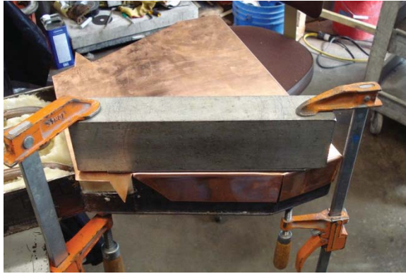
Figure C.11: Seating of flashing prior to drilling for screw holes.
