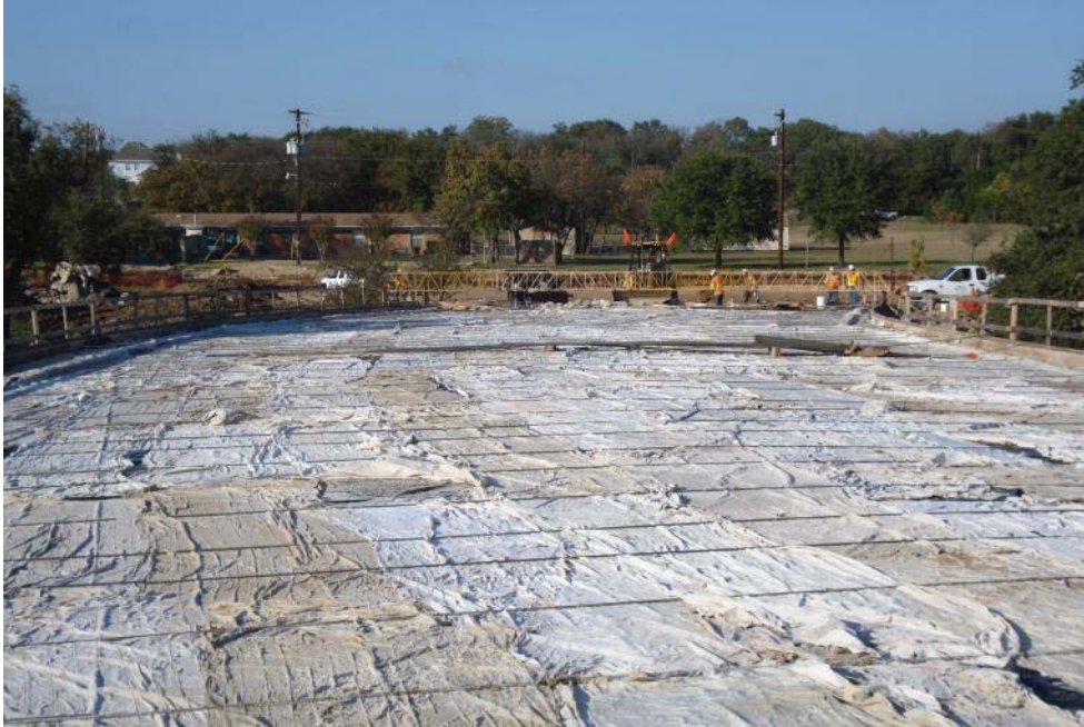
Figure 7.23: Curing method for Georgetown bridge deck winter pour.
