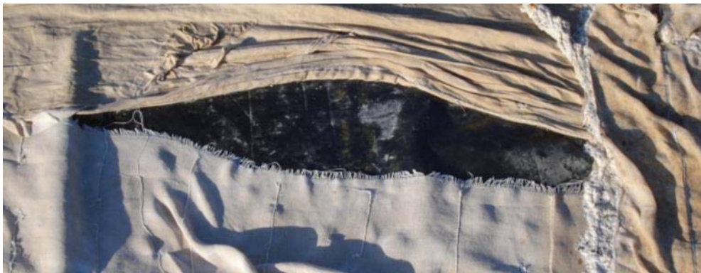
Figure 7.24: Black plastic under curing blanket at Georgetown winter pour.
