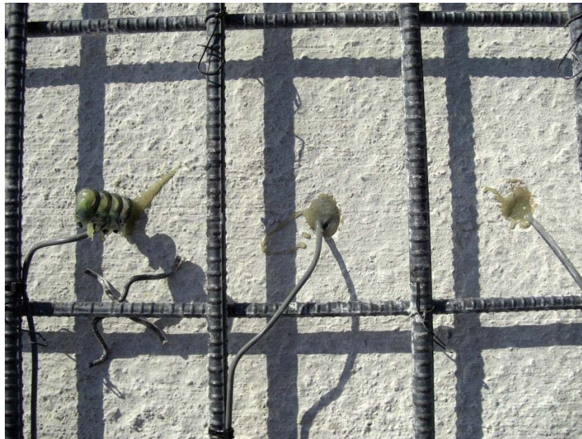
Figure 7.42: Completed bridge deck instrumentation.
