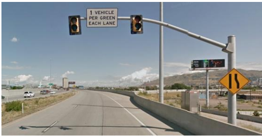
Figure 5.7 Large Traffic Signal
