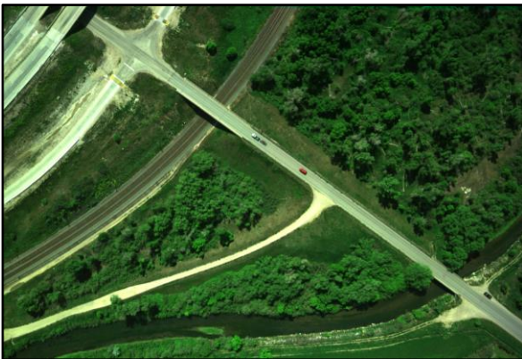
Figure 2.5 Aerial Photography No.1
