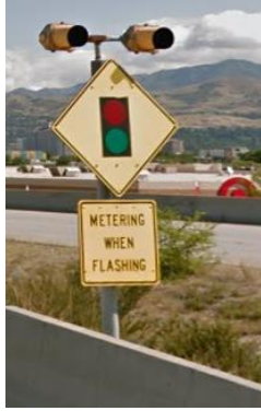
Figure 5.5 Small Traffic Signal
