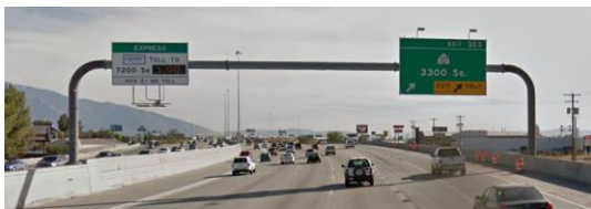
Figure 5.3 Overhead Traffic Sign
