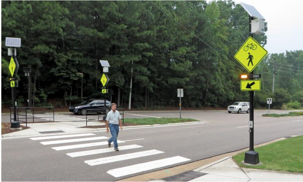
Figure 12. Flashing Crossing Signage (Source: Texas Transportation Institute)
