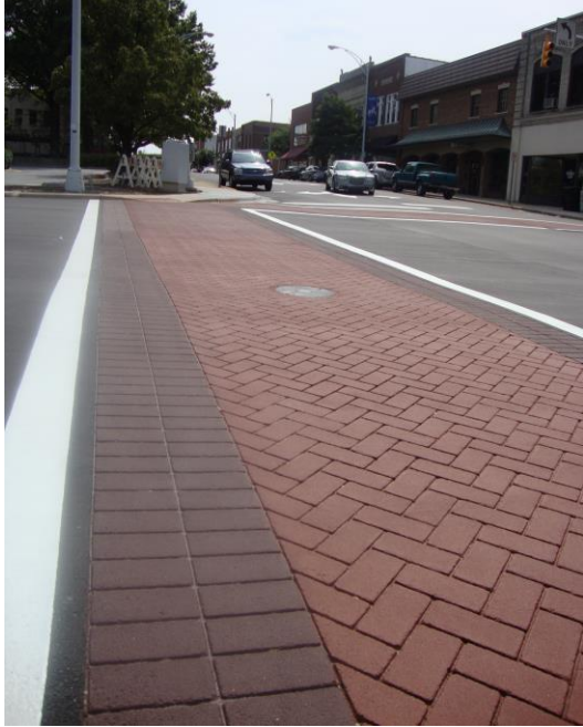
Figure 10. Stamped Asphalt Crosswalk (Source: myaspaltdr.files.wordpress.com )
