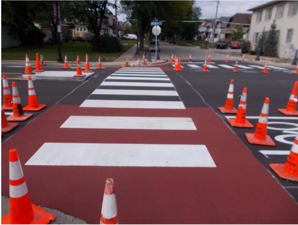
Figure 8. High-Contrast Crosswalk Paint (Source: www.urbanmilwaukee.com )
