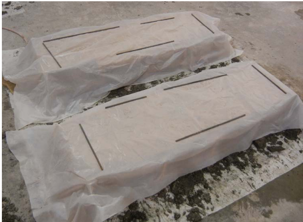
Figure 3-11: Slabs covered in burlap and wrapped in plastic
