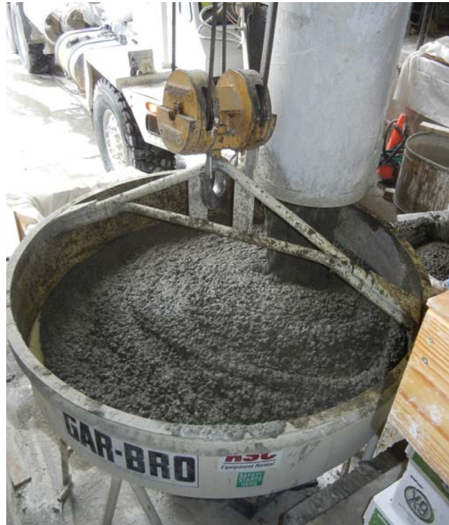
Figure 3-9: Placing concrete into placement bucket
