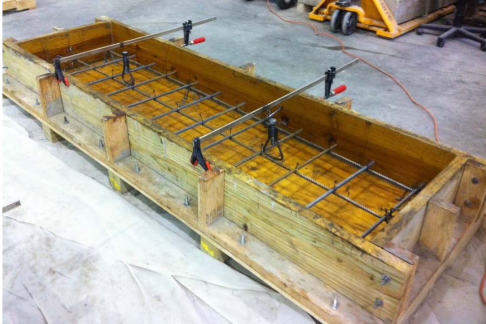
Figure 3-7: Tied reinforcing bars for a slab element
