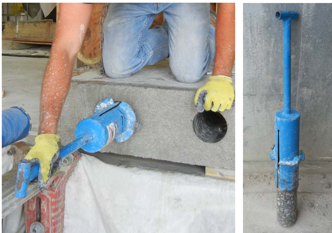
Figure 3-15: Retrieving cores using a coresnap
