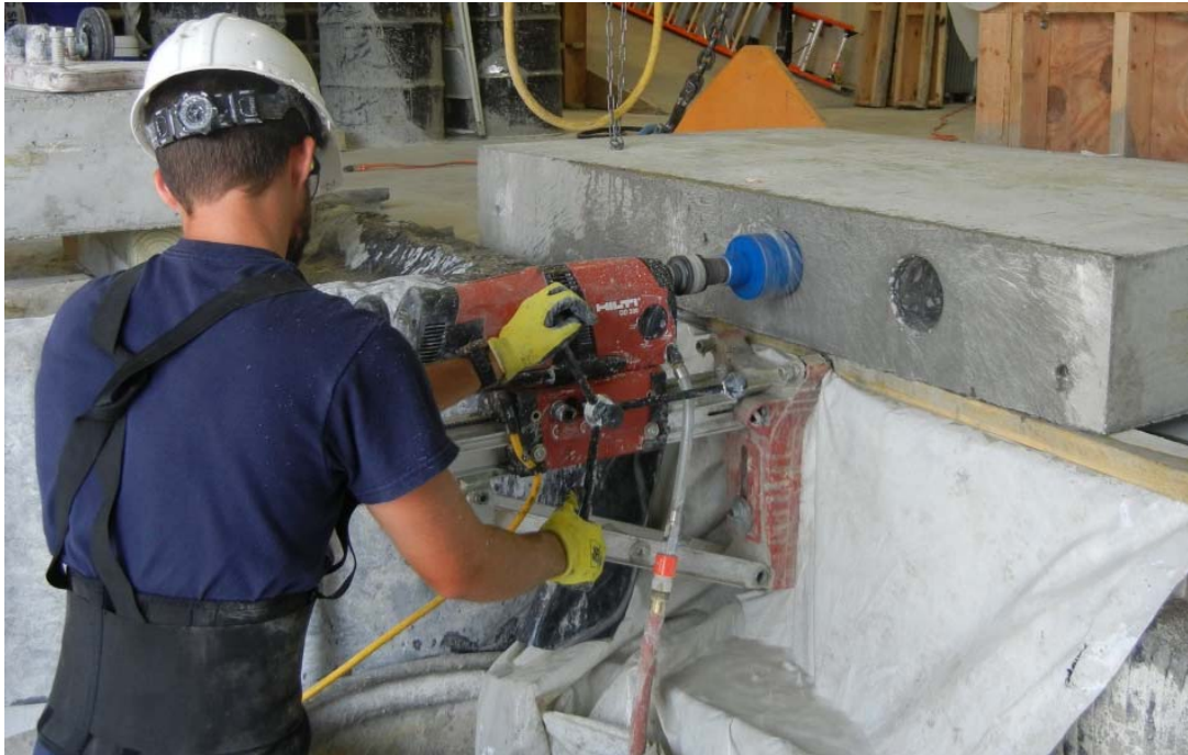
Figure 3-14: Core rig mounted to AU Structural Engineering Laboratory loading dock
