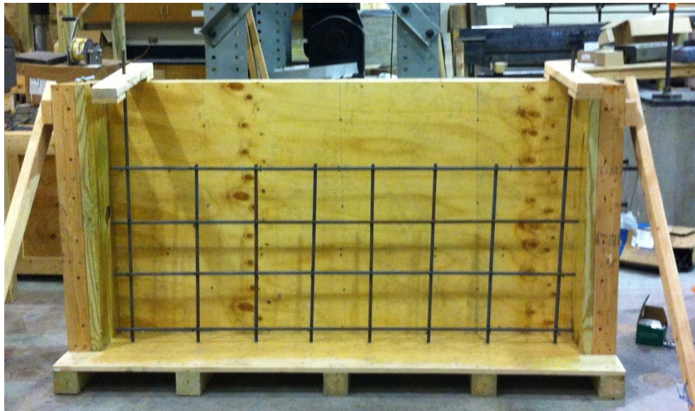
Figure 3-8: Tied reinforcing bars for the wall element
