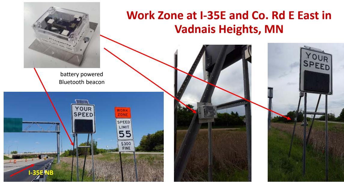
Figure 3-9 Installation of a Bluetooth Beacon at a Highway Work Zone
