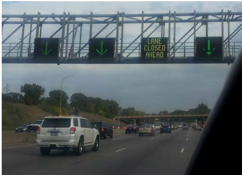
Figure 1-1. Gantry displaying ILCS messages.
