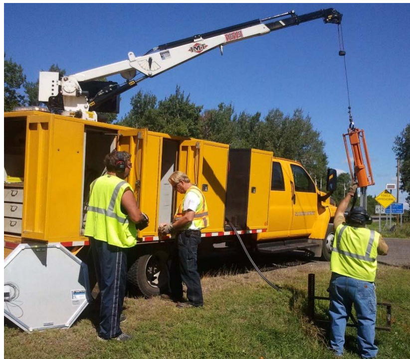
Figure 45: Installing the STOP sign posts using the Sign Shop utility truck.
