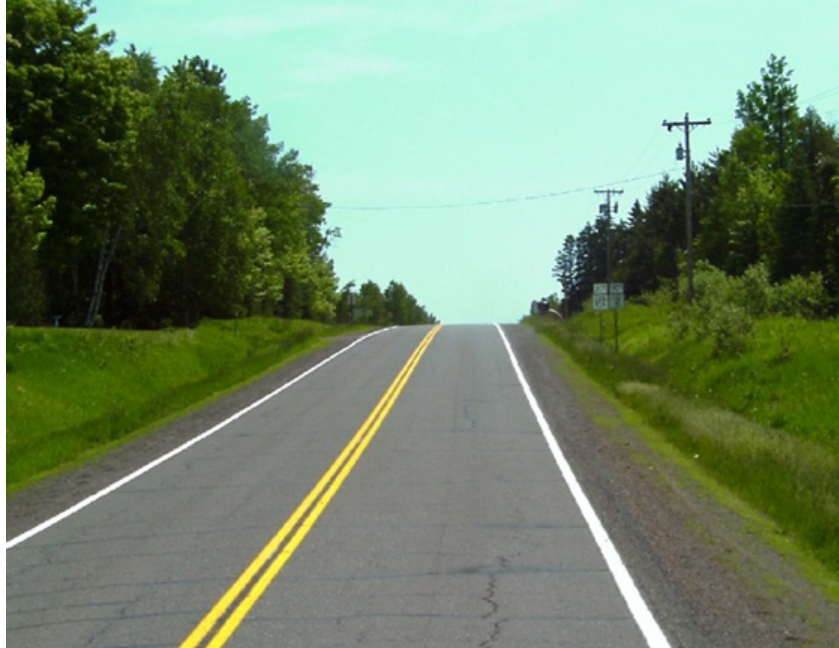
Figure 2: Sight restriction of the intersection for drivers traveling from the west side of Lismore Road.
