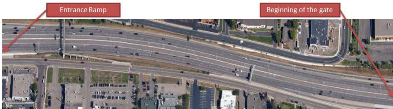
Figure 106. Test Site on I-394
