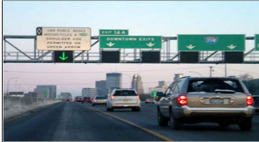
Figure 3. Interstate 35W, Minneapolis, MN
