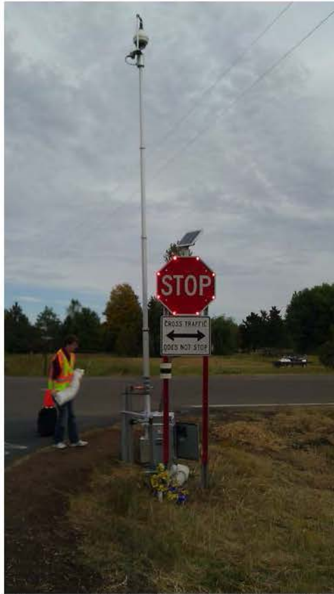
Figure 3.9 Flashing LED Stop Sign and Video Equipment on Southeast Corner of Study Site
