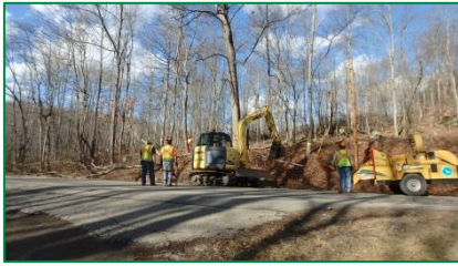
Photograph 105. Ground crew and excavator loading the Vermeer BC 1500 brush chipper.
