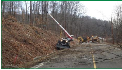
Photograph 102. All-terrain tree trimmer followed by excavator, brush chipper, and ground crew.
