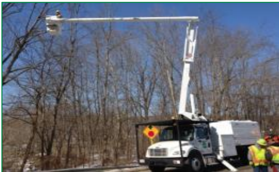
Photograph 94. ODOT employee removing branches to the branch collar while using a forestry bucket truck.
