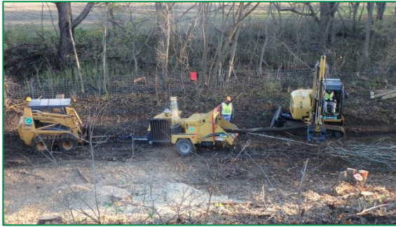
Photograph 108. Ground crew and excavator loading brush chipper with material. The material was cut by a ground crew of sawyers.
