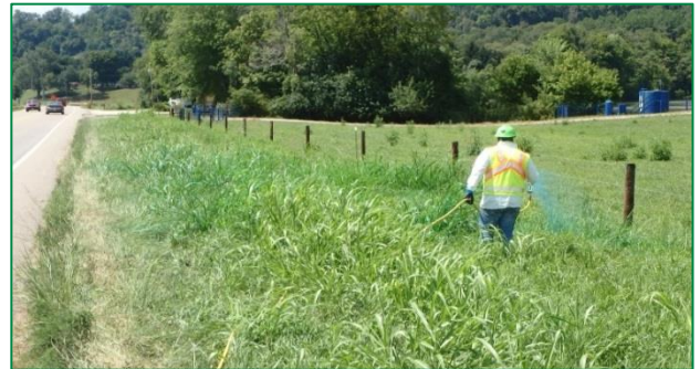
Photograph 38. ODOT employee applying directed herbicide to Johnsongrass in test plots. The herbicide application was timed for when the Johnsongrass is days to weeks away from fully opening its flowers.
