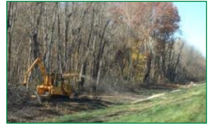
Photograph 101. ODOT employee performing debris clean-up using Bandit chipper following all-terrain tree trimmer.
