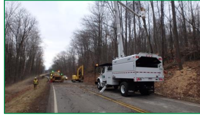
Photograph 103. Forestry bucket truck followed by excavator, brush chipper, and ground crew.
