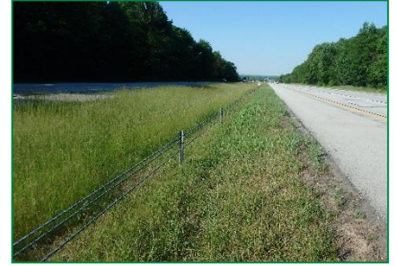
Photograph 17. Turf height is controlled as a result of properly timed Plateau® application. The cable rail is visible, although no mechanical clearing has been performed.
