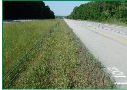
Photograph 16. Turf height is controlled as a result of properly timed Embark® application. The cable rail is visible, although no mechanical clearing has been performed.
