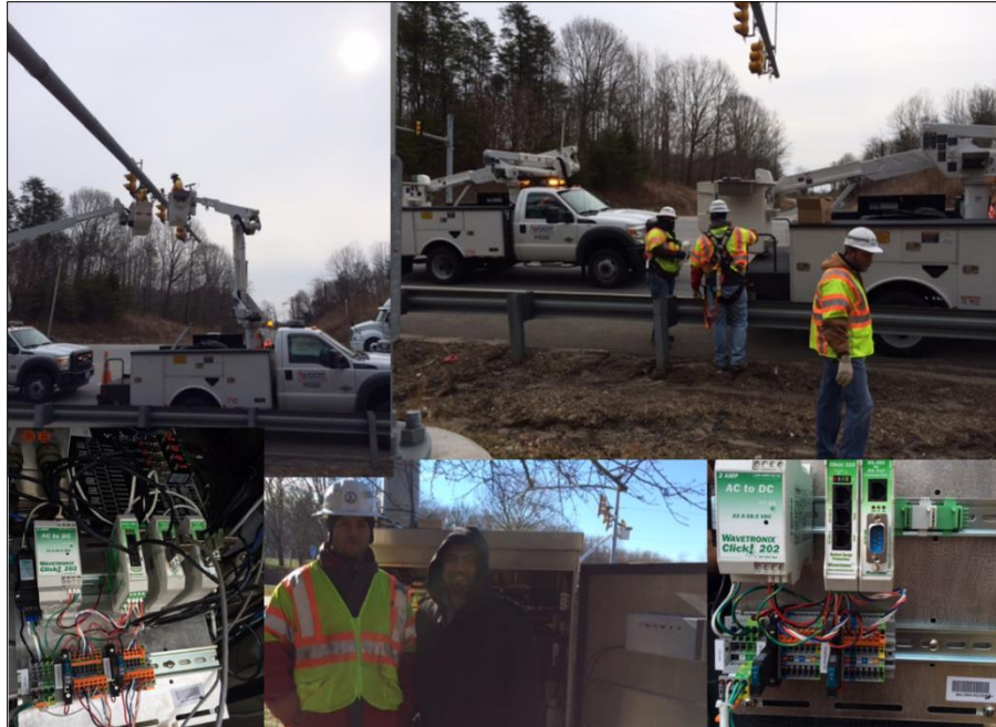
Figure 10. Field Installation of Data Collection System
