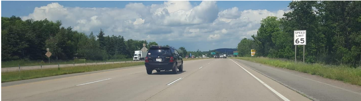
Figure 39: Bordered contrast markings on NB US-51
