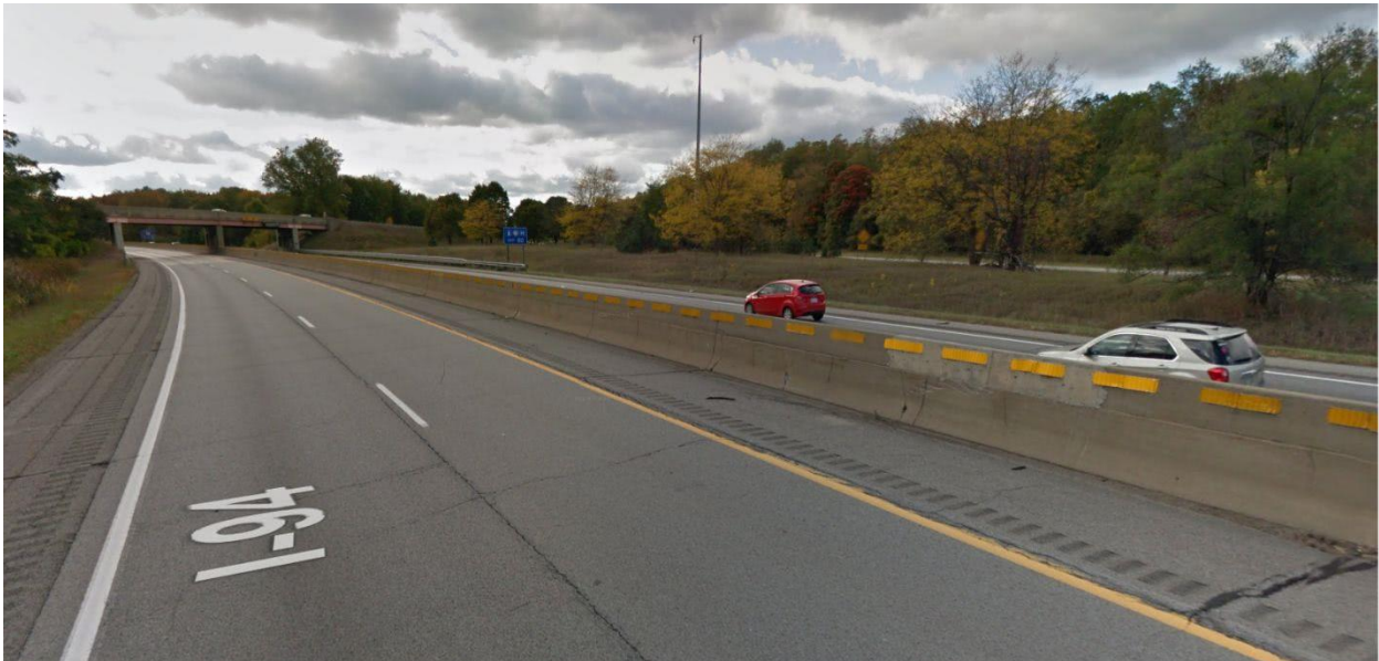
Figure 27: 3M LDS barrier side mount reflectors on EB I-94, west of I-94BL, Kalamazoo, Michigan (Image courtesy of Google Street View)
