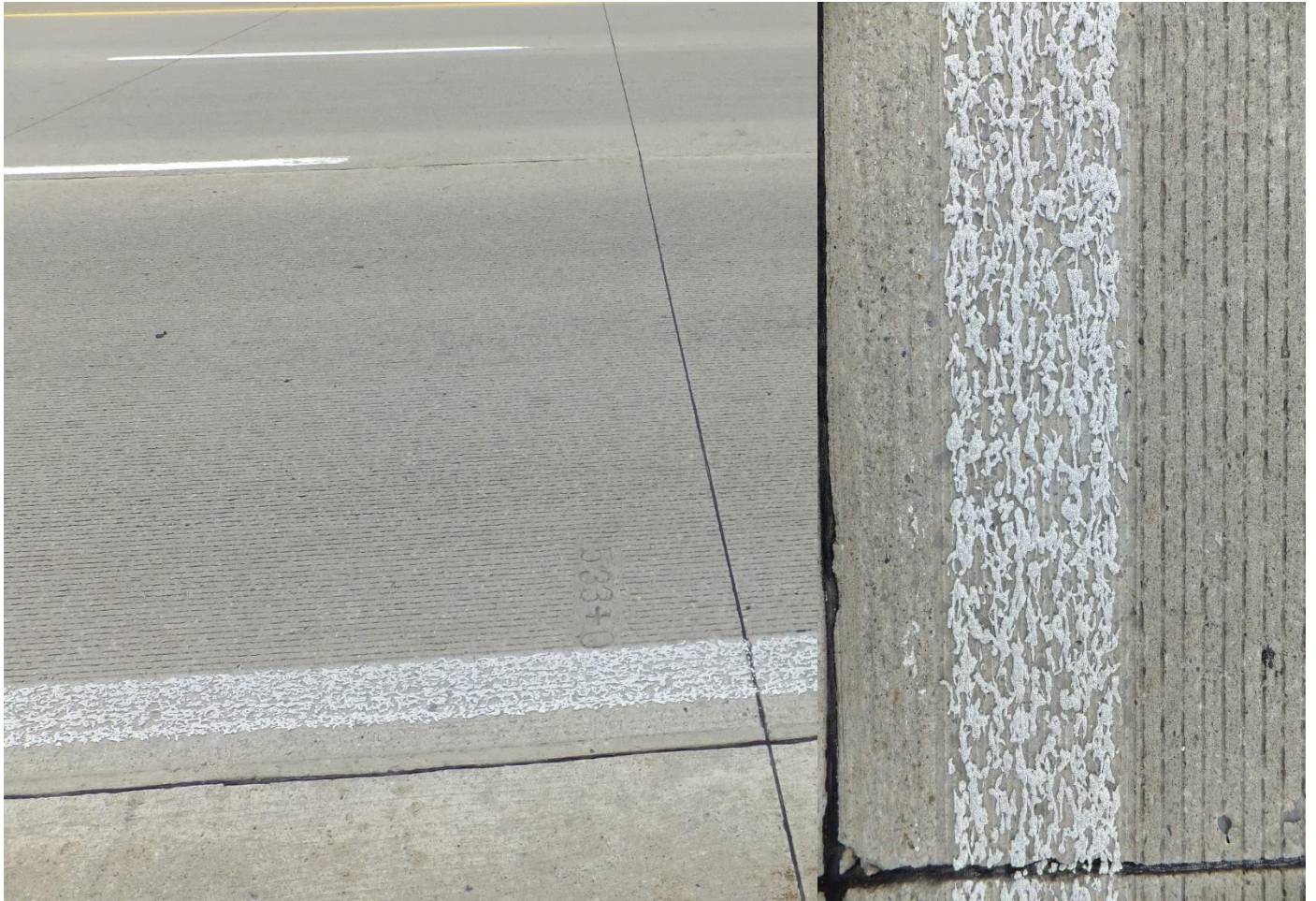
Figure 31: Profiled (splatter) Methyl Methacrylate edge line, from side and top
