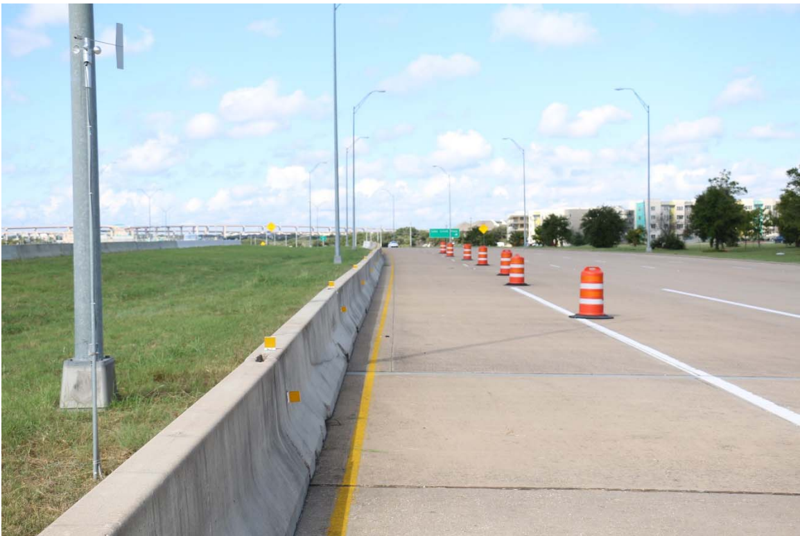
Figure 7.4 Additional highway barriers and road hazard barrels
