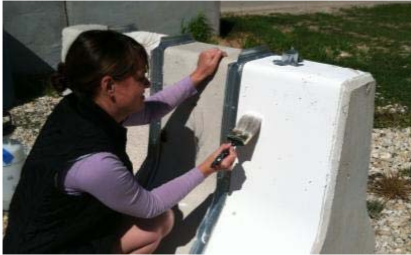
Figure 3.5 Application of the white paint
