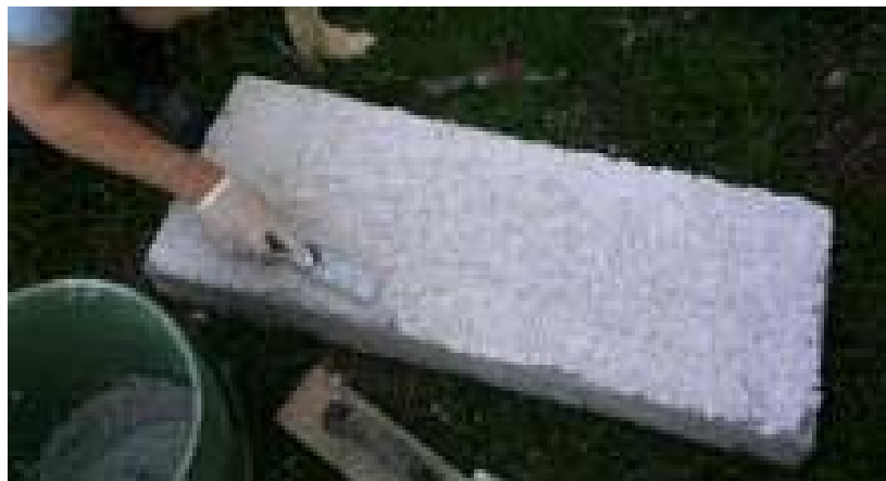
Figure 3.4 Application of the photocatalytic stucco
