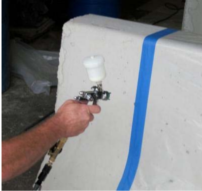
Figure 3.6 Clear paint 1 application by sprayer
