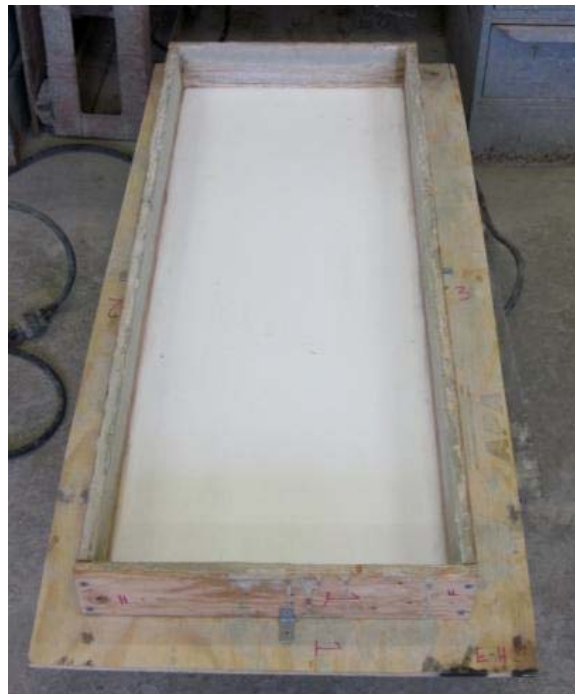
Figure 3.2 Completed slab formwork
