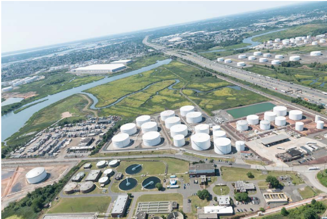
Figure 34 3D Dense Reconstruction Site 1
