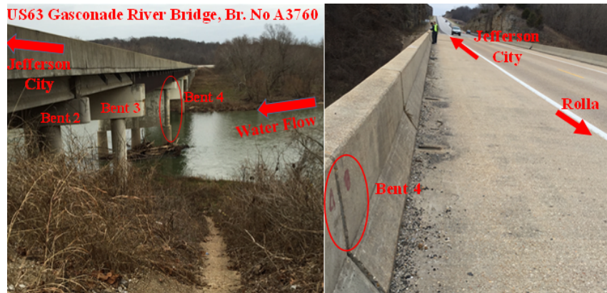
Figure 5.21. The US Highway 63 Gasconade River Bridge.
