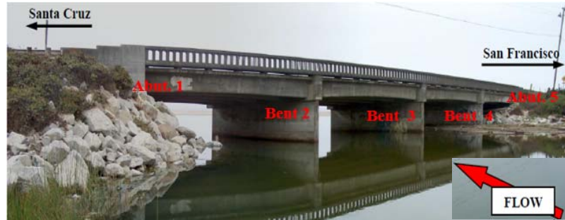
Figure 5.12. State Highway 1 Bridge over Waddell Creek, CA.
