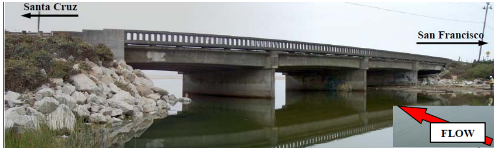
Figure 2.5. State Hwy1 Bridge over the Waddell Creek.
