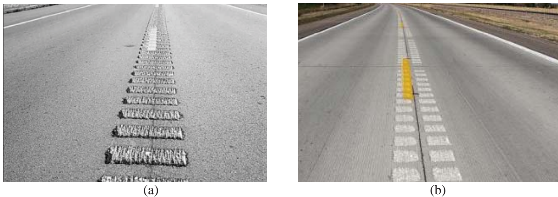
Figure 1-4. CLRSs in Nebraska: (a) old design; (b) current design.
