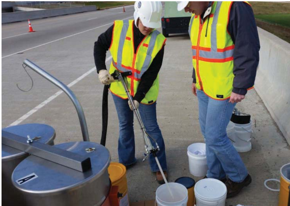
Figure 5.5 Ensuring proper mixing of sealer components.
