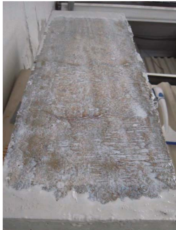
Figure 2.17 Sealer applied to cracked control Specimen No. 22.
