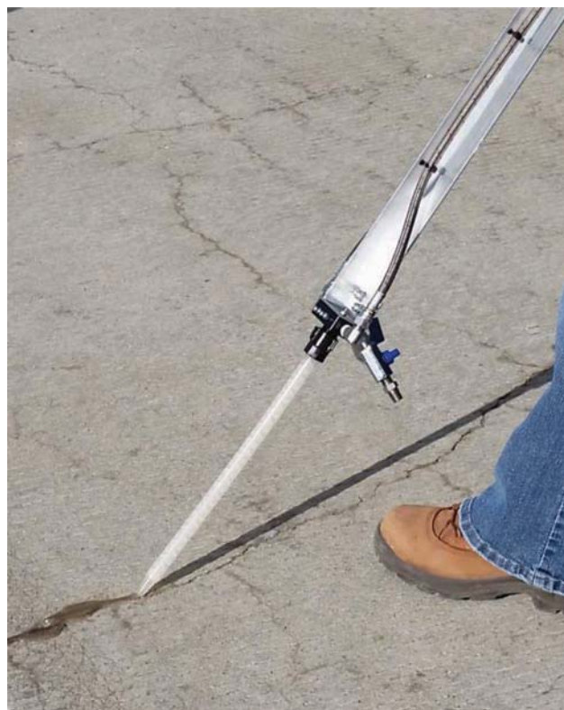
Figure 5.2 Applicator wand and attached static mixer.
