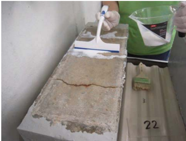
Figure 2.16 Applying deck sealer to cracked control Specimen No. 22.
