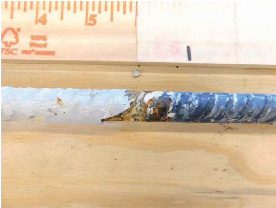
Figure 3.15 Corrosion on top half of increment No. 1.
