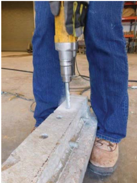
Figure 3.21 Drilling specimens to collect chloride test samples.
