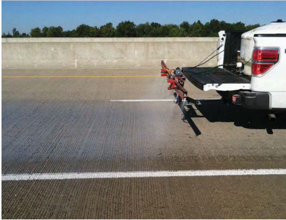
Figure 5.8 Application of MasterProtect H 400 using truck-mounted sprayer bar.
