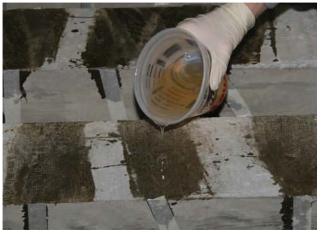
Figure 2.9 Installation of crack sealers (Lyrenmann, 2011).
