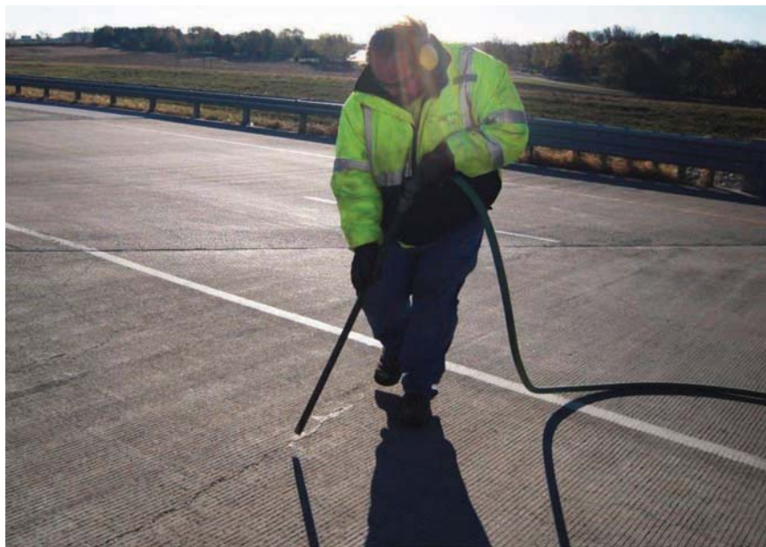
Figure 5.3 Using compressed air to clean the cracks.
