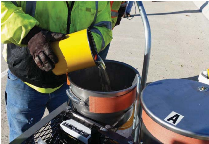
Figure 5.4 Pouring sealer components into reservoir tanks.
