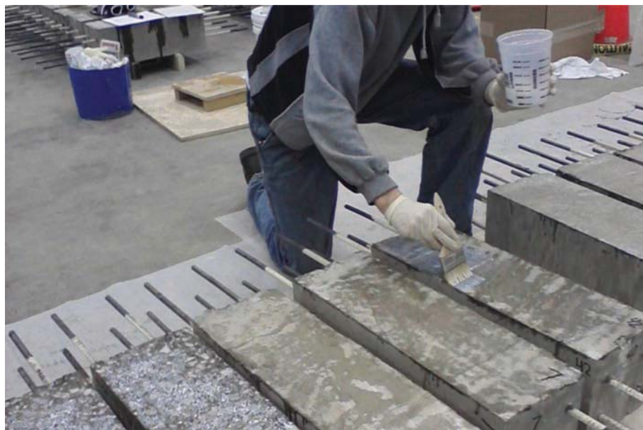
Figure 2.10 Application of deck sealers (Lyrenmann, 2011).
