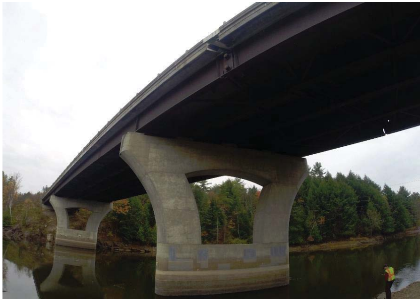
Figure 23: Bents, deck and beams
