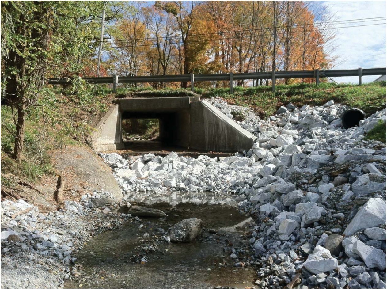
Figure 4.34 Vt. Rte. 30 Pawlet Br. #78 - REPAIRED Wing Wall reconstruction, $80,000
