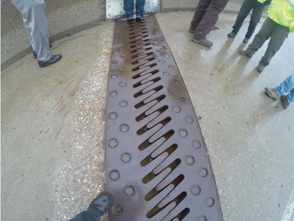
Figure 5.17 Finger expansion joint on US 2 Lamoille River Crossing Bridge
