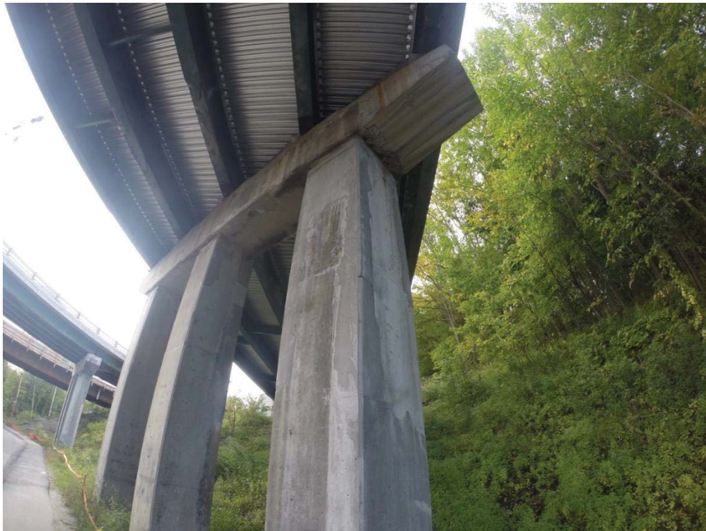
Figure 5.49 Pier on I-89 Waterbury Overpass Bridge with patch repairs
