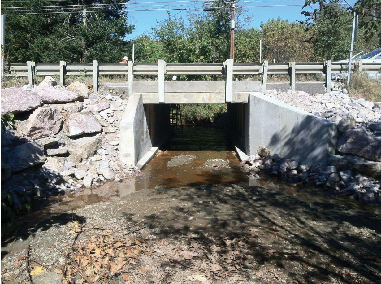
Figure 4.28 Vt. Rte. 12 Berlin Br. #70 - REPAIRED Head Wall/Wing Wall Reconstruction, $150,000
