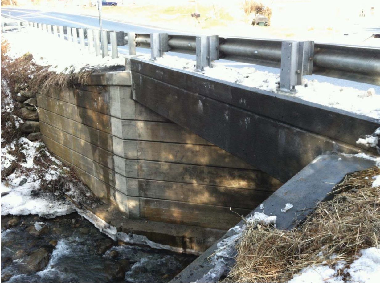
Figure 4.42 Vt. Rte. 113 Vershire Br. #11 - REPAIRED Deck/Wing Wall Repairs, $150,000
