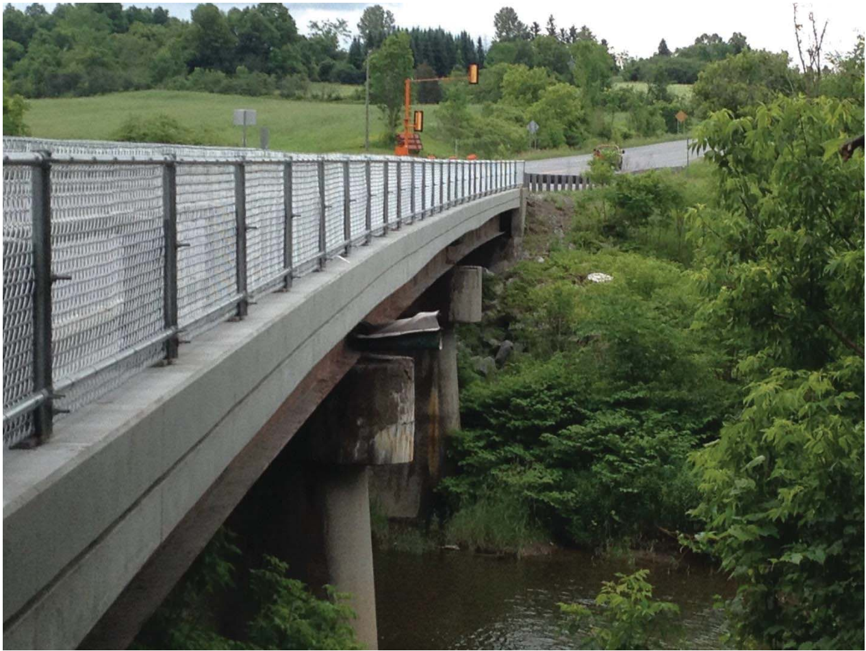
Figure 4.6 US 7 New Haven Br. #129 – REPAIRED Fascia/Curb Reconstruction, $350,000
