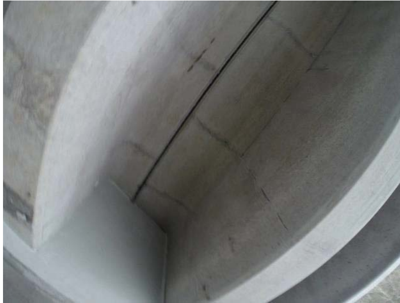
Figure 5.43 Girders have multiple cracks in top flanges, Stowe Rte 100 Gold Brook Crossing Bridge
