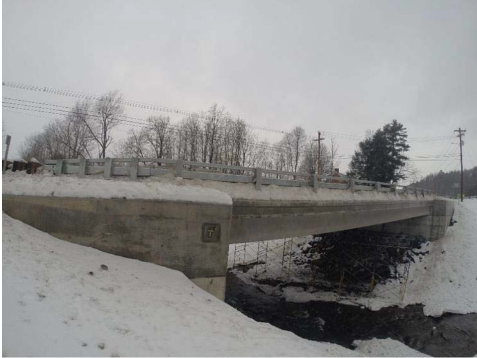
Figure 5.41 Stowe Rte 100 Gold Brook Crossing Bridge
