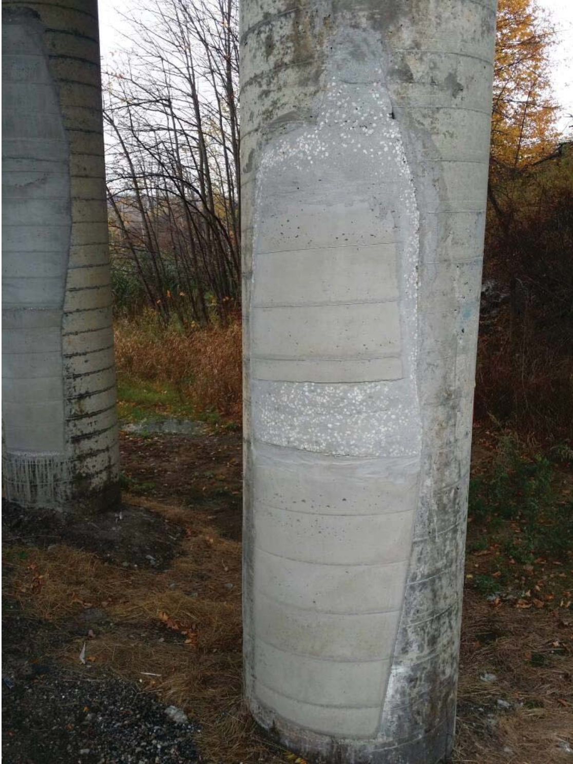
Figure 5.26 Large column patch repair #2 on Williston I-89 Oak Hill Rd Underpass Bridge
