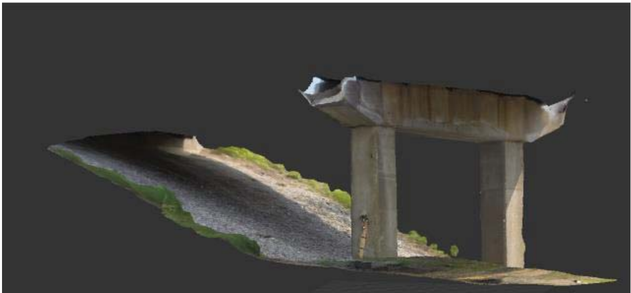
Figure 5.4 Photogrammetric 3-D point cloud rendering of Swanton I 89 overpass bridge pier from right side.
