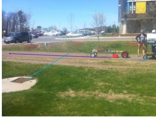
Figure 45 The photo of the test site with underground sewer
