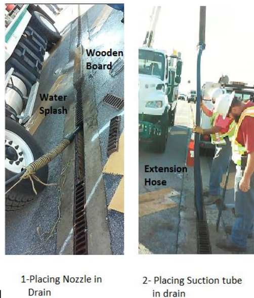
Figure 9- Use of sewer cleaner in cleaning trench drains
