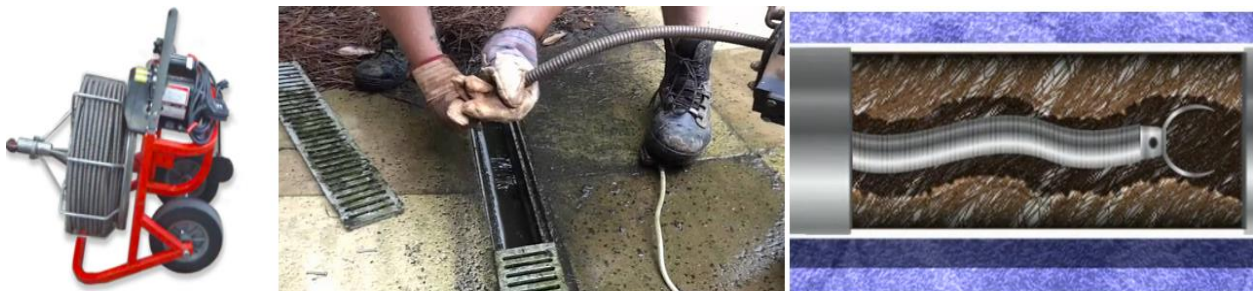
Figure 18. Cleaning a Trench Drain by a Mechanical Drain Cleaner
