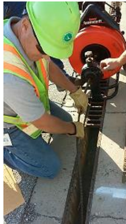
Figure 8- Use of mechanical drain in cleaning trench drains
