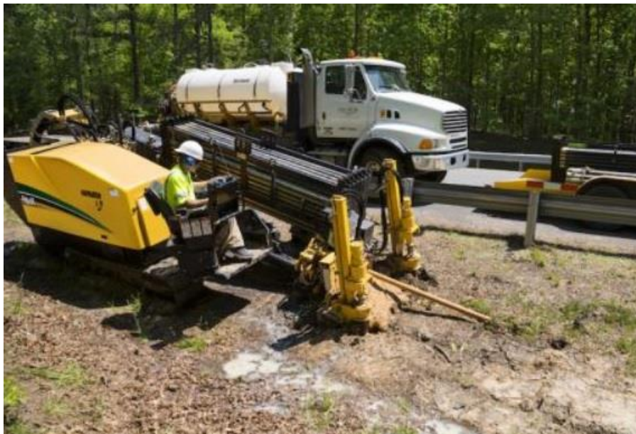
Figure 22. Installing pipes using a HDD rig
