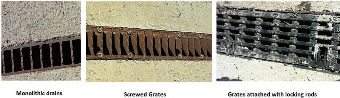
Figure 4. Different style of drains
