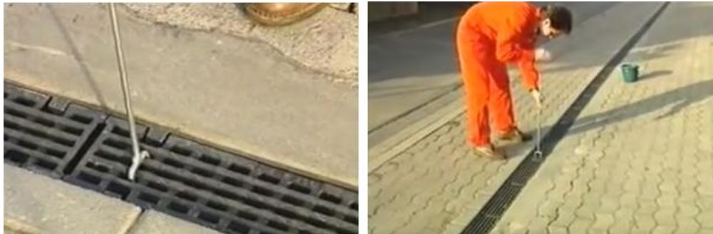
Figure 5. Tool to remove grates attached with locking rods
