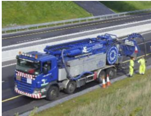
Figure 20. Cleaning a Trench Drain by a Vactor-jet
