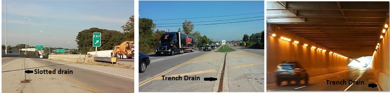
Figure 2- Various installations of trench and slotted drains in Franklin County, Ohio
