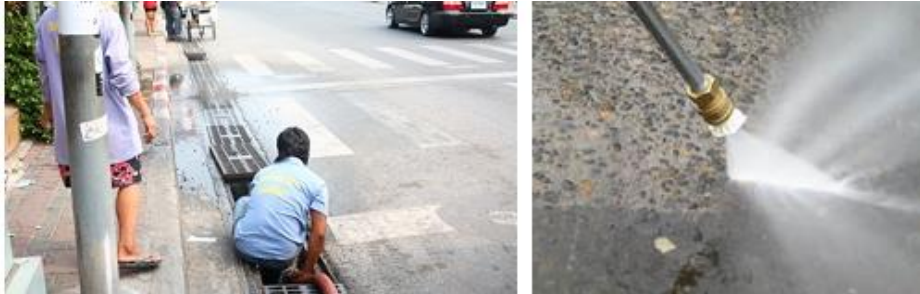
Figure 17. Cleaning Trench Drains by Flushing with Water
