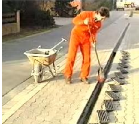
Figure 16. Manual Cleaning of Trench drains
