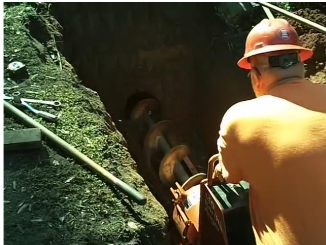
Figure 23. Horizontal Auger Boring
