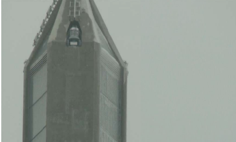
Figure 1.19: Ice accumulation on pylon glazing February 24, 2011
