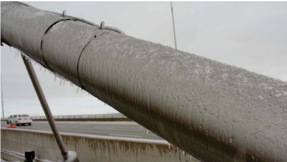
Figure 1.12: Frozen Rivulets and bare metal on the west side of stays February 22, 2011
