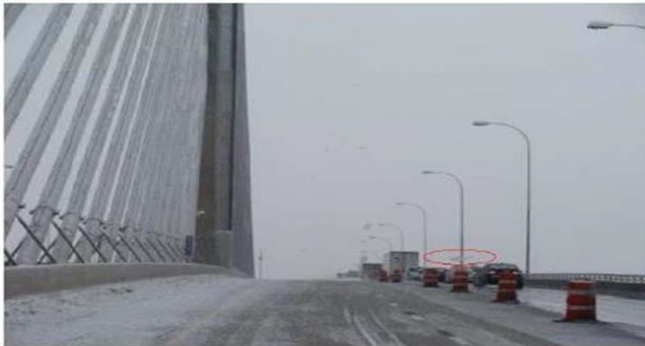
Figure 1.5: Large Piece of Ice Almost Hitting a Car
