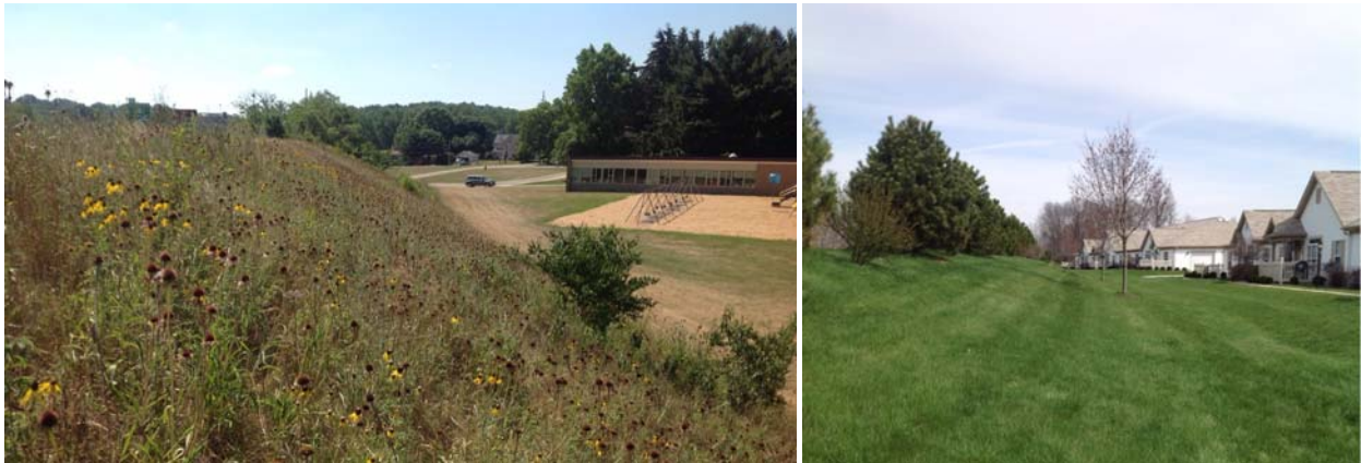
Figure 3-1: Sample Earthen Berms (Left: Site 45, STA-77 SB & Right: Site 10, TRU-11 NB)
