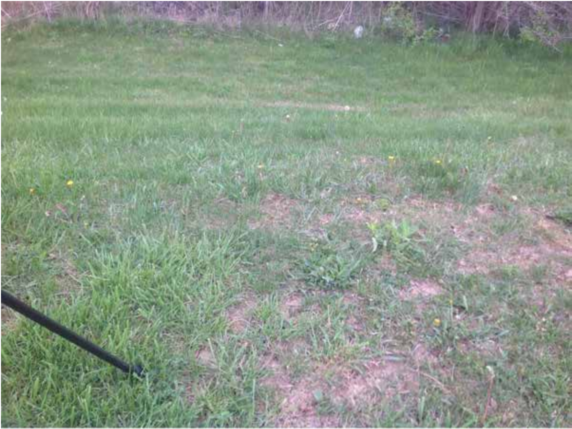
Site 23: FRA-270 EB, Parsons Ave (Enchanted Estates), Looking at Noise Berm Vegetation
