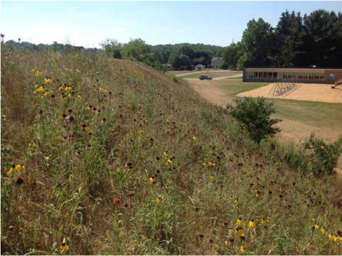
Site 45: STA-77 SB, 38th St NW (Little Eagle Kindergarten), Looking along Noise Berm Eastern Slope
