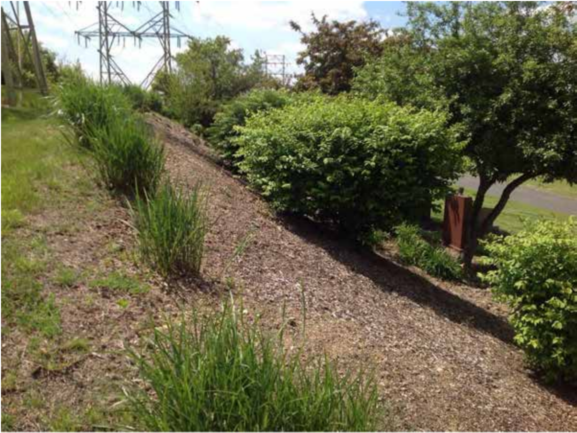
Site 32: SUM-277 WB, Glenmount Ave (Holy Cross Cemetery), Looking along Noise Berm Northern Slope
