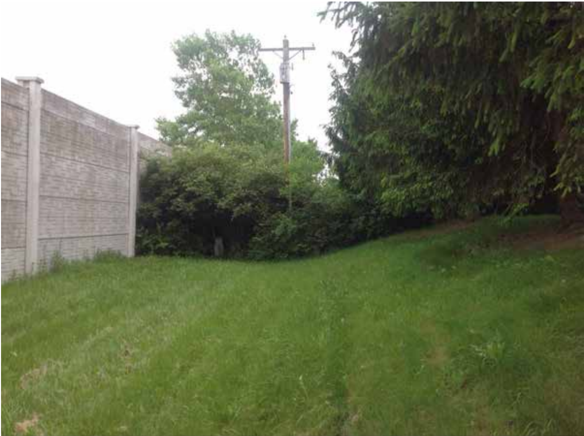
Site 38: MIA-75 SB (Woodlawn Dr), Looking at Structural Wall
