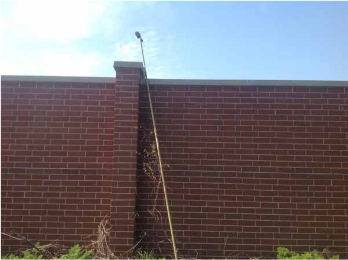
Site 22: MAD-70 EB, Karen Drive, Looking at Meter A
