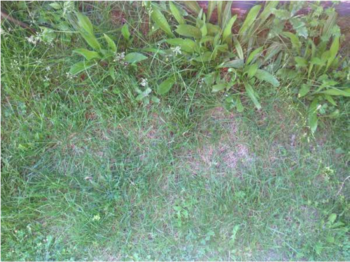
Site 37: FRA-71 NB (Grand Stand Drive Community), Looking at Noise Berm Vegetation
