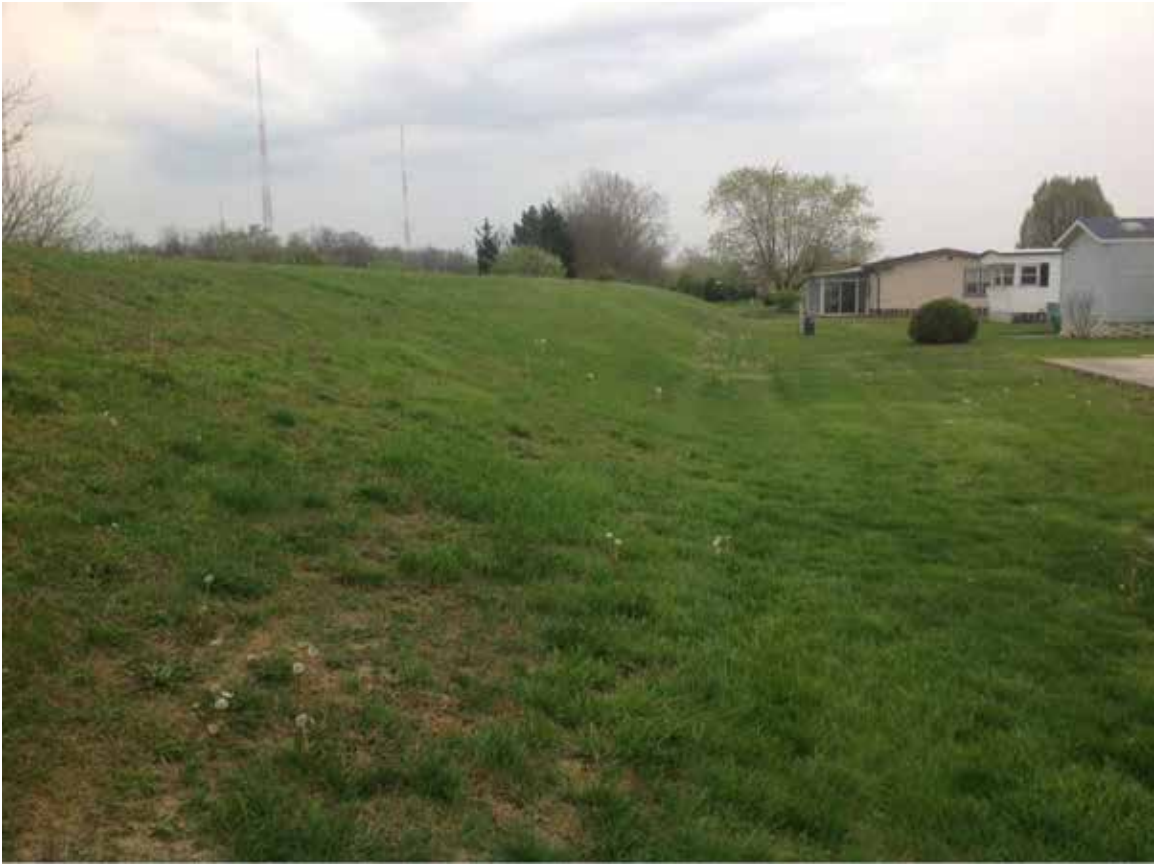
Site 23: FRA-270 EB, Parsons Ave (Enchanted Estates), Looking along Noise Berm Southern Slope
