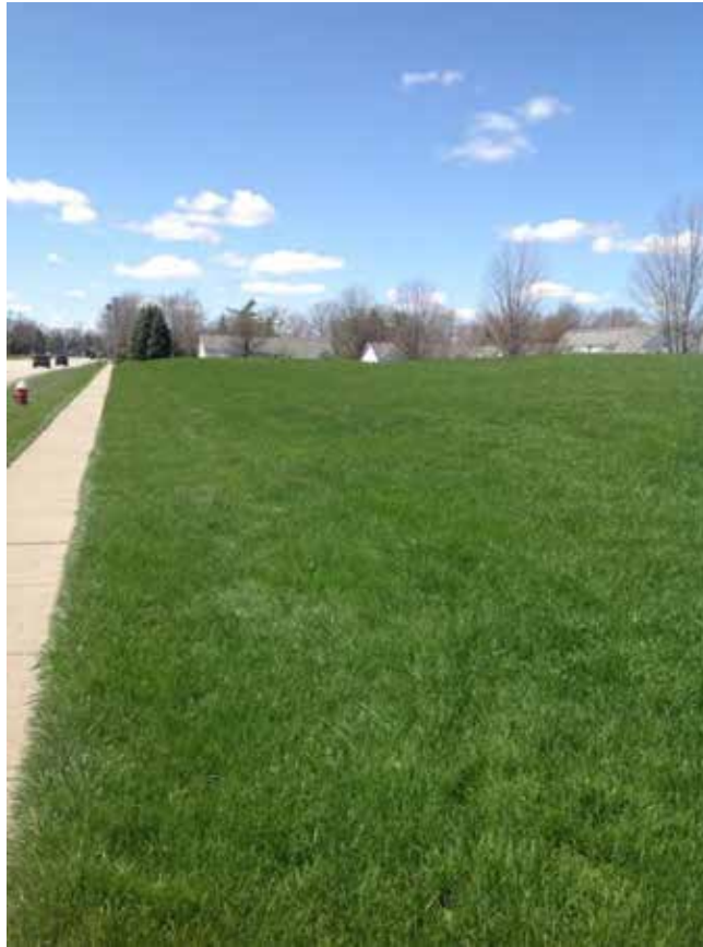
Site 8: LUC-Heatherdown Blvd WB, Looking along Noise Berm Western Slope
