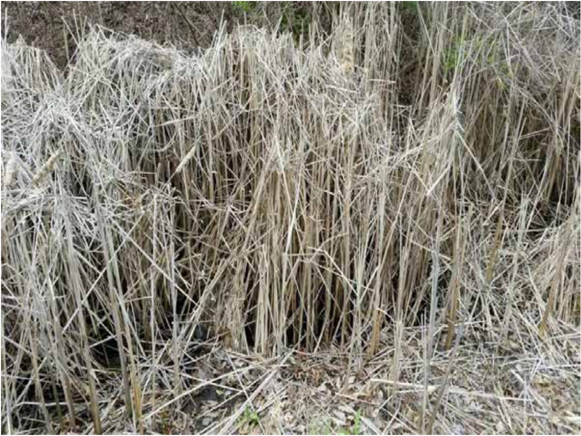
Site 12: POR-76 EB, Rest Area (between Porter and Alliance Roads), Looking along Noise Berm Southern Slope
