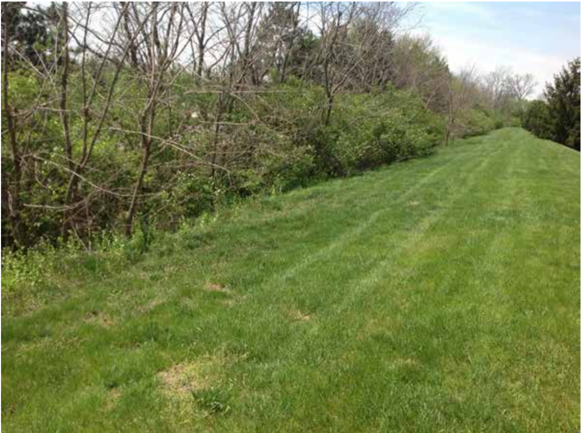
Site 20: MON-675 SB, Bigger Rd (Piper Landing Apartments), Looking along Noise Berm Eastern Slope
