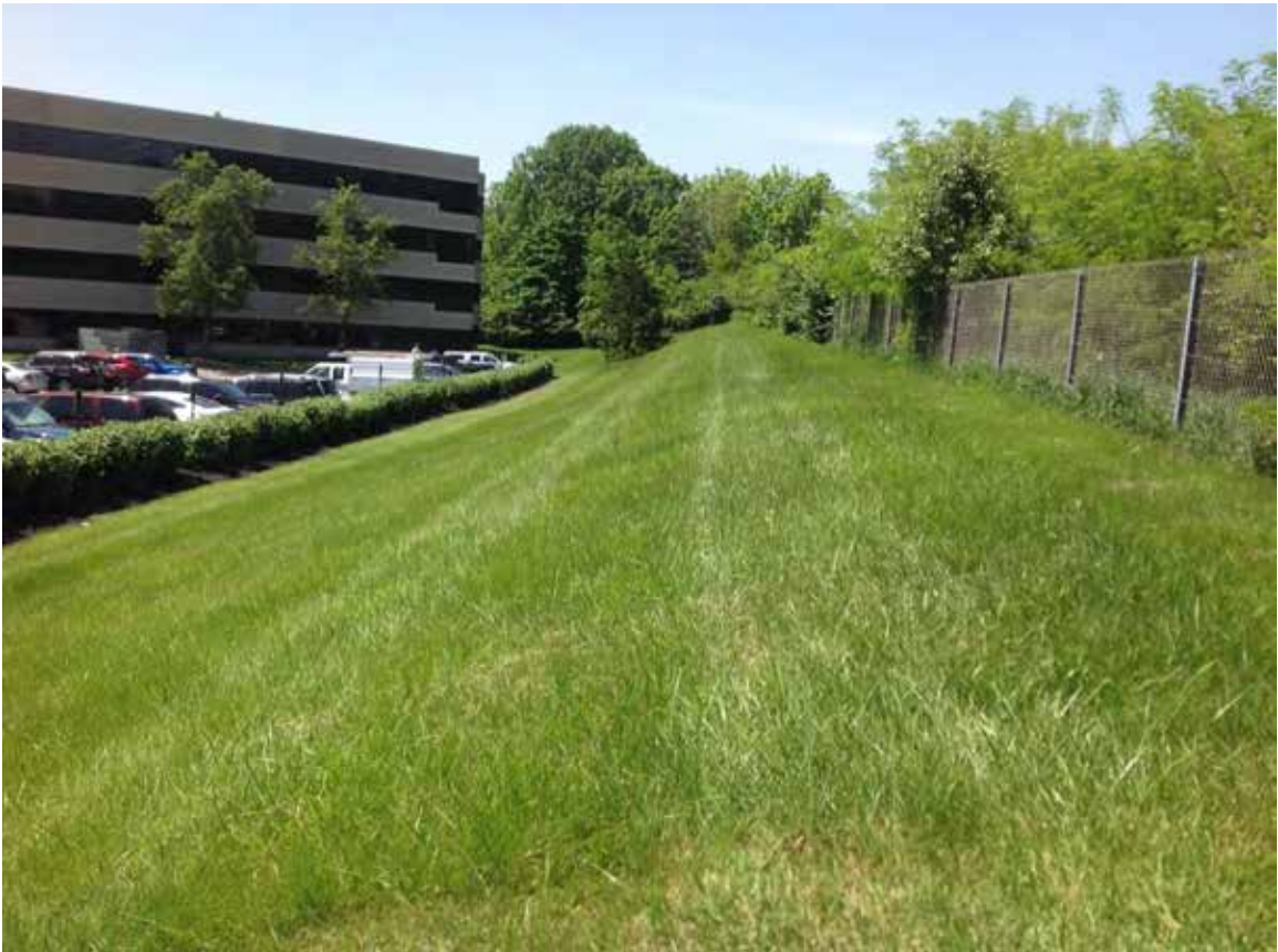
Site 35: HAM-71 NB, Governor's Hill Dr, Looking along Noise Berm Eastern Slope
