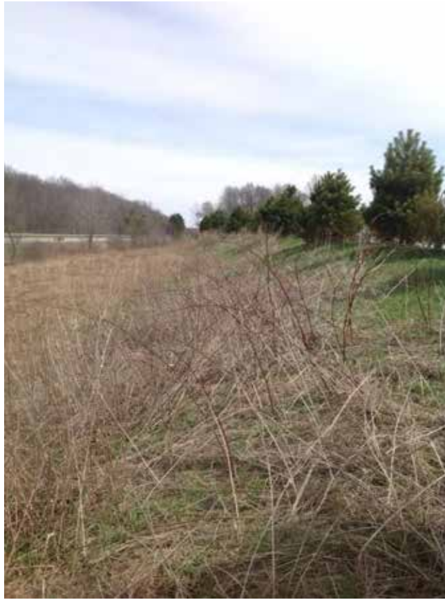
Site 10: TRU-SR11 NB, Avalon Creek Blvd, Looking along Noise Berm Western Slope
