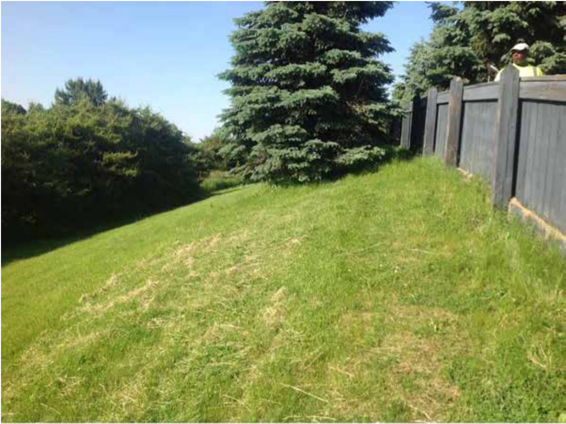
Site 37: FRA-71 NB (Grand Stand Drive Community), Looking along Noise Berm Western Slope
