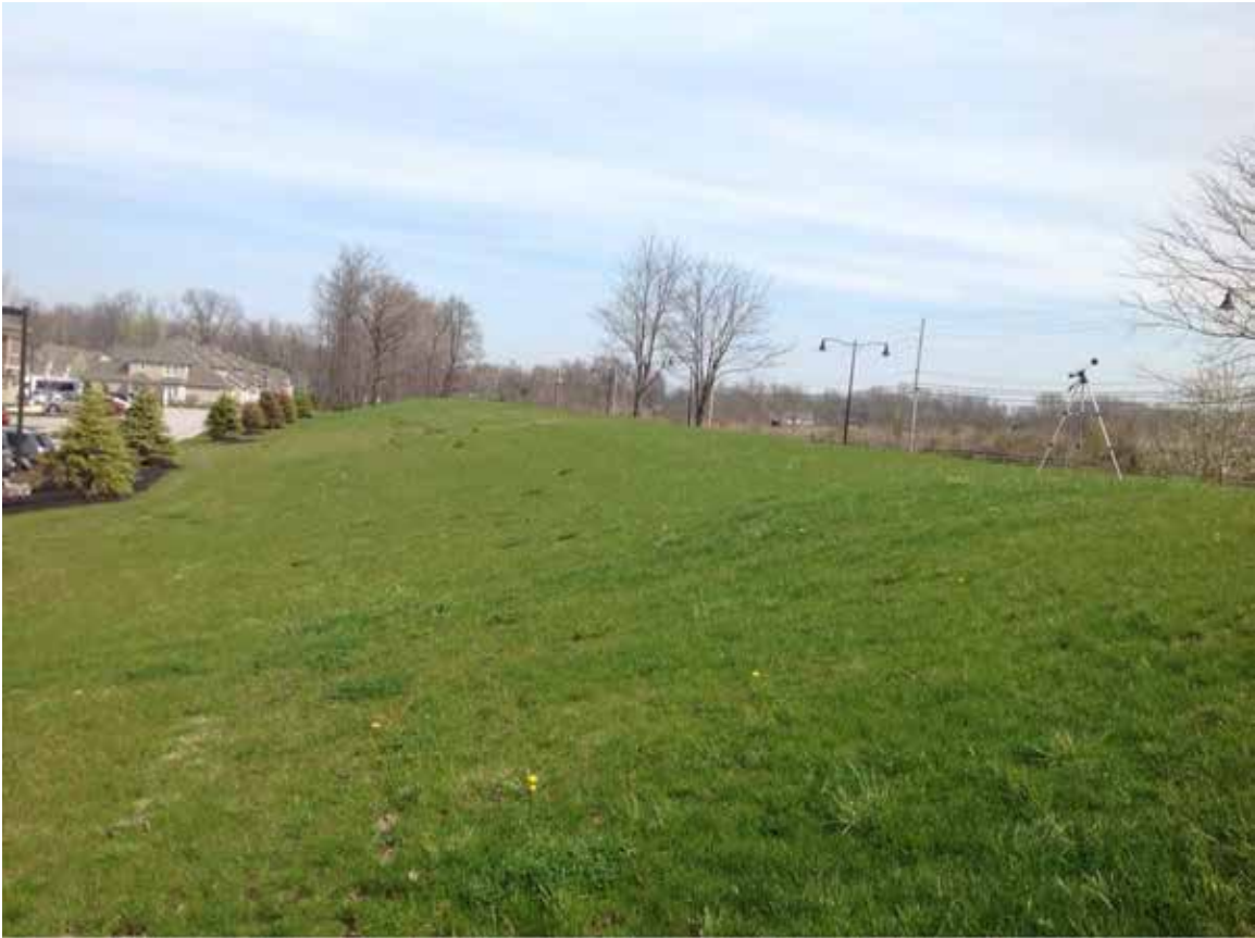
Site 16: LAK-SR615 SB, Emeritus at Newell Creek Condos, Looking along Noise Berm Western Slope
