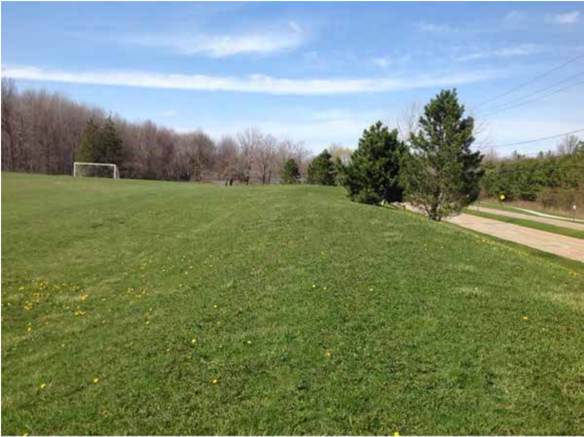
Site 18: CUY-SR91 SB, N, Commons Blvd (Progressive Bldg), Looking along Noise Berm Western Slope
