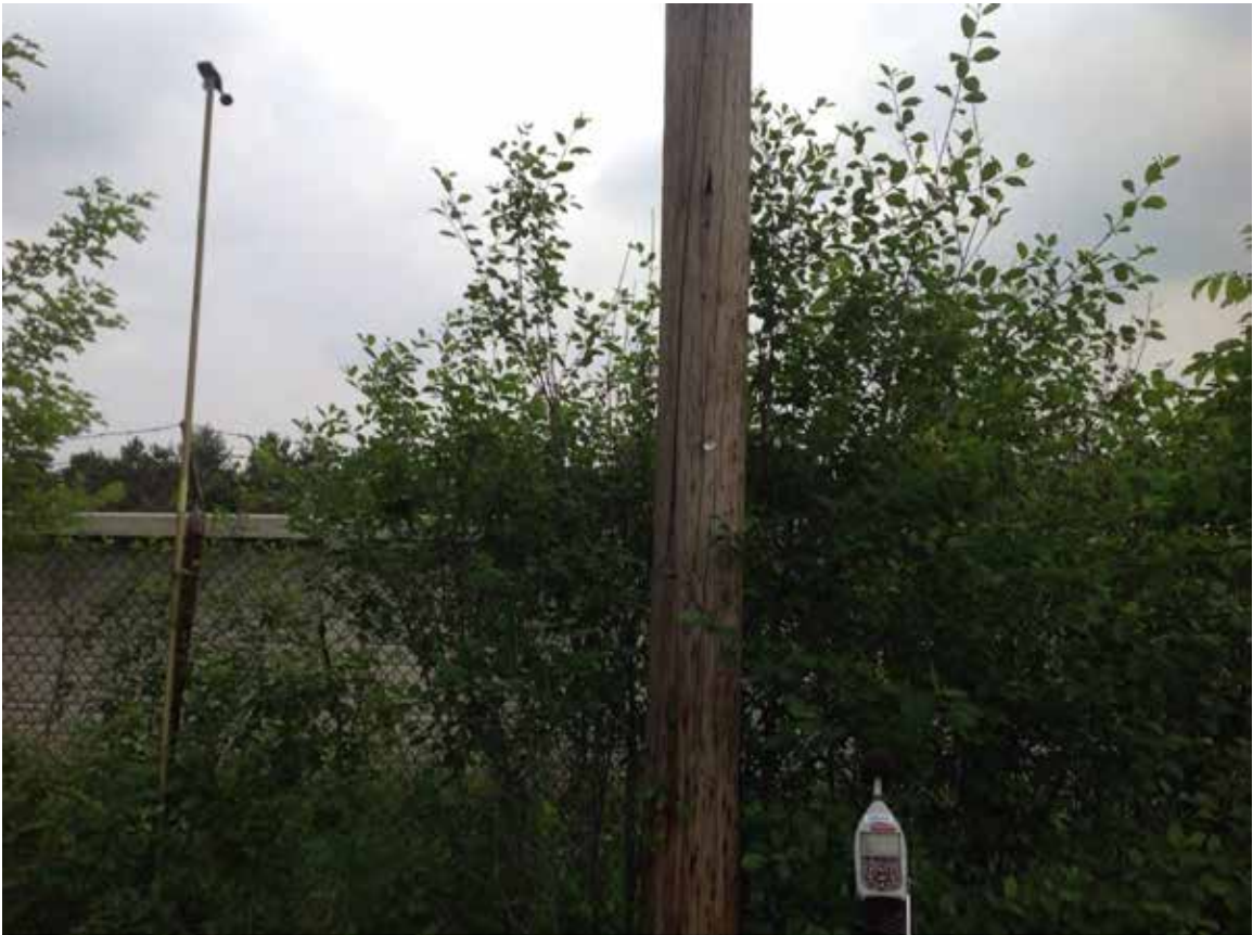
Site 41: CUY-80 EB, Surrey Circle, Looking at Meter B
