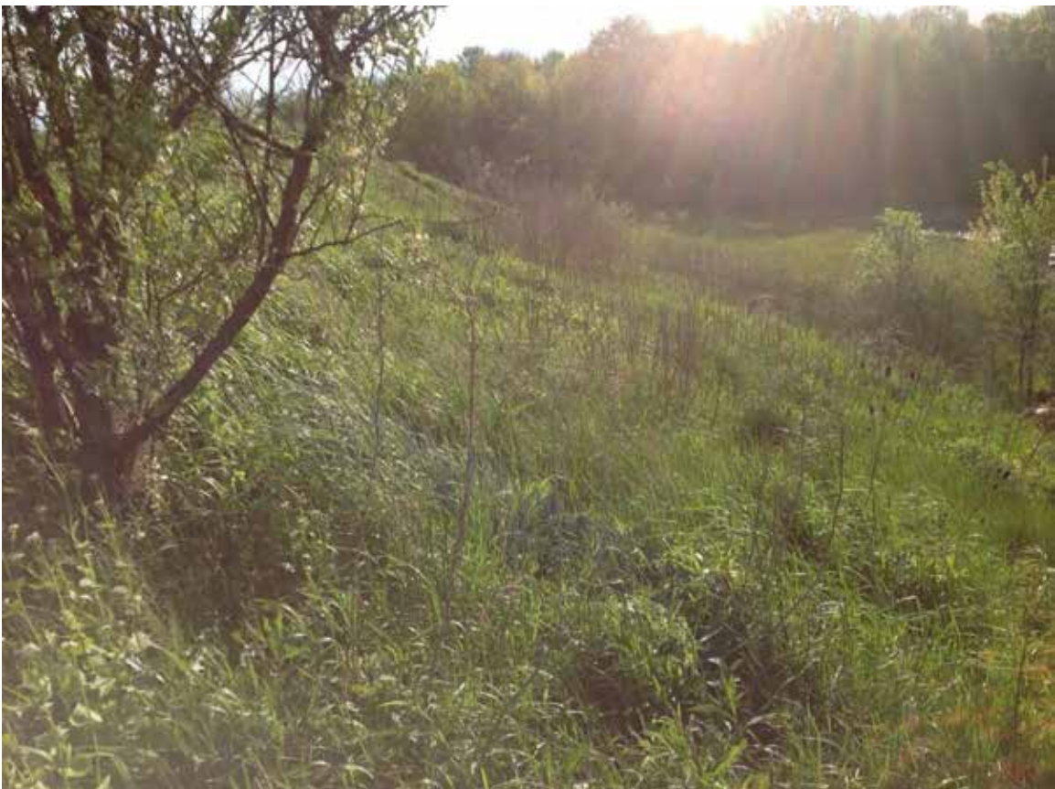
Site 30: ASH-71 SB, Ashland Country Rd 1095, Looking along Noise Berm Southern Slope
