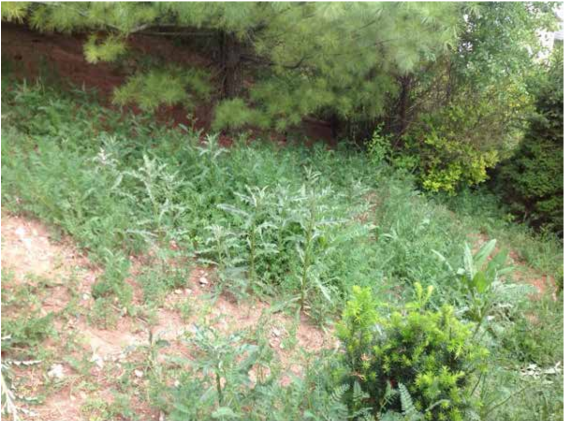
Site 40: LOG-SR33 EB, Shawnee Trace, Looking along Noise Berm Western Slope
