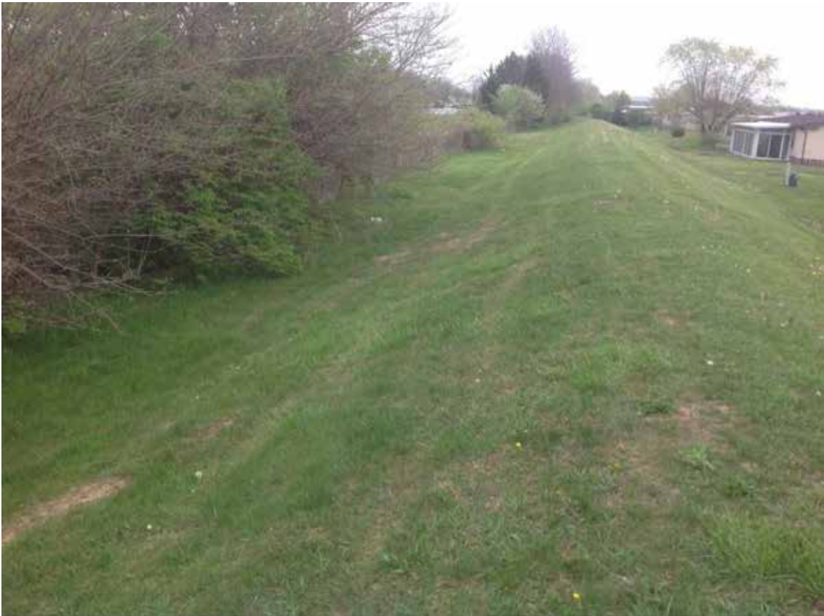
Site 23: FRA-270 EB, Parsons Ave (Enchanted Estates), Looking along Noise Berm Northern Slope
