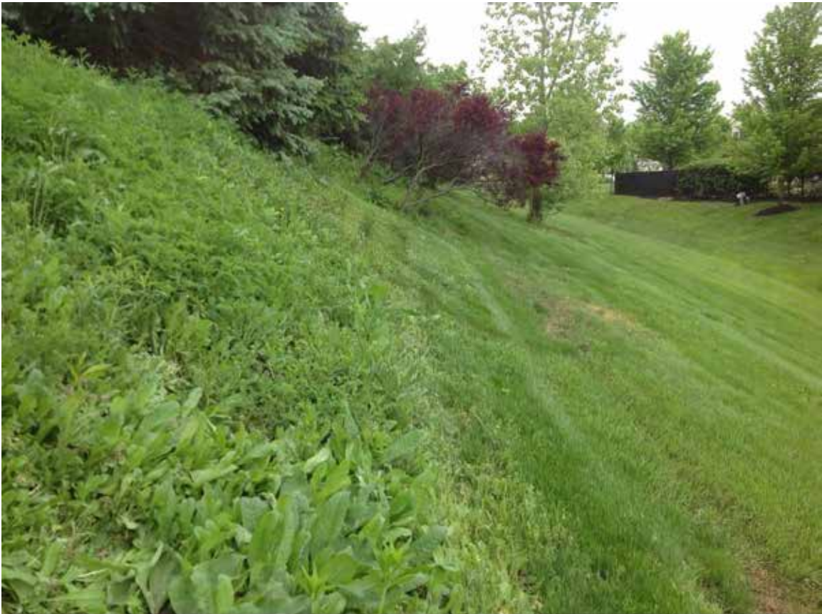
Site 1: DEL-71 NB, Tournament Drive, Looking along Noise Berm Eastern Slope
