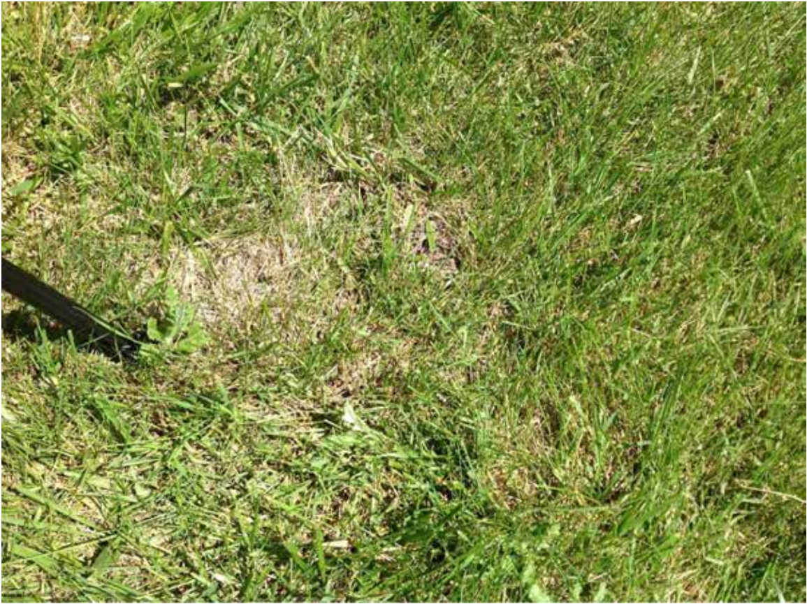
Site 35: HAM-71 NB, Governor's Hill Dr, Looking at Noise Berm Vegetation
