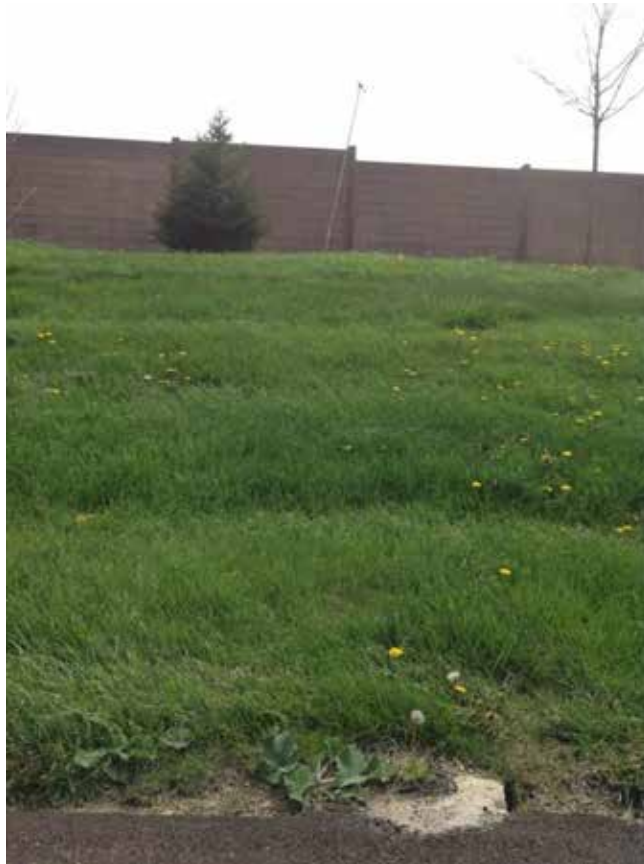
Site 21: MON-675SB, Bigger Rd (Carriage Trace Apartments), Looking at Structural Wall
