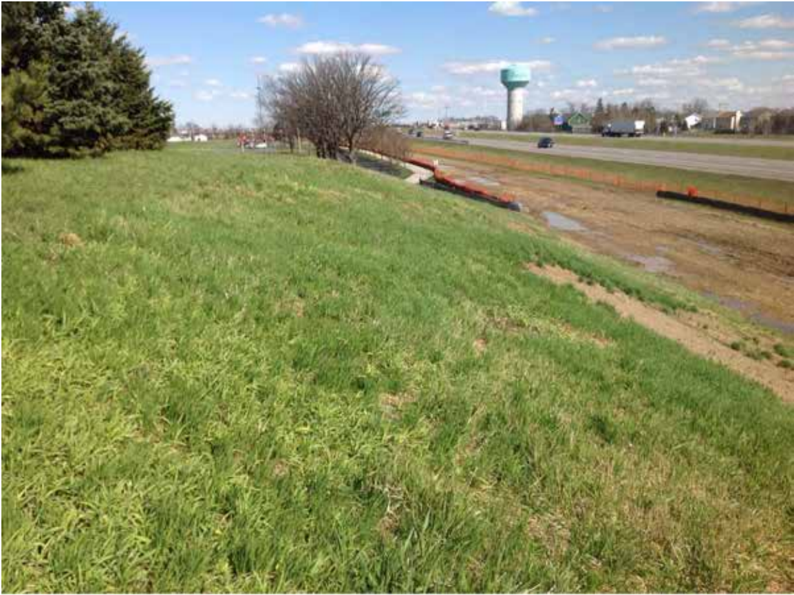
Site 9: WOO-475 NB, Ft, Meigs Rd (Rivercrest Park), Looking along Noise Berm Eastern Slope
