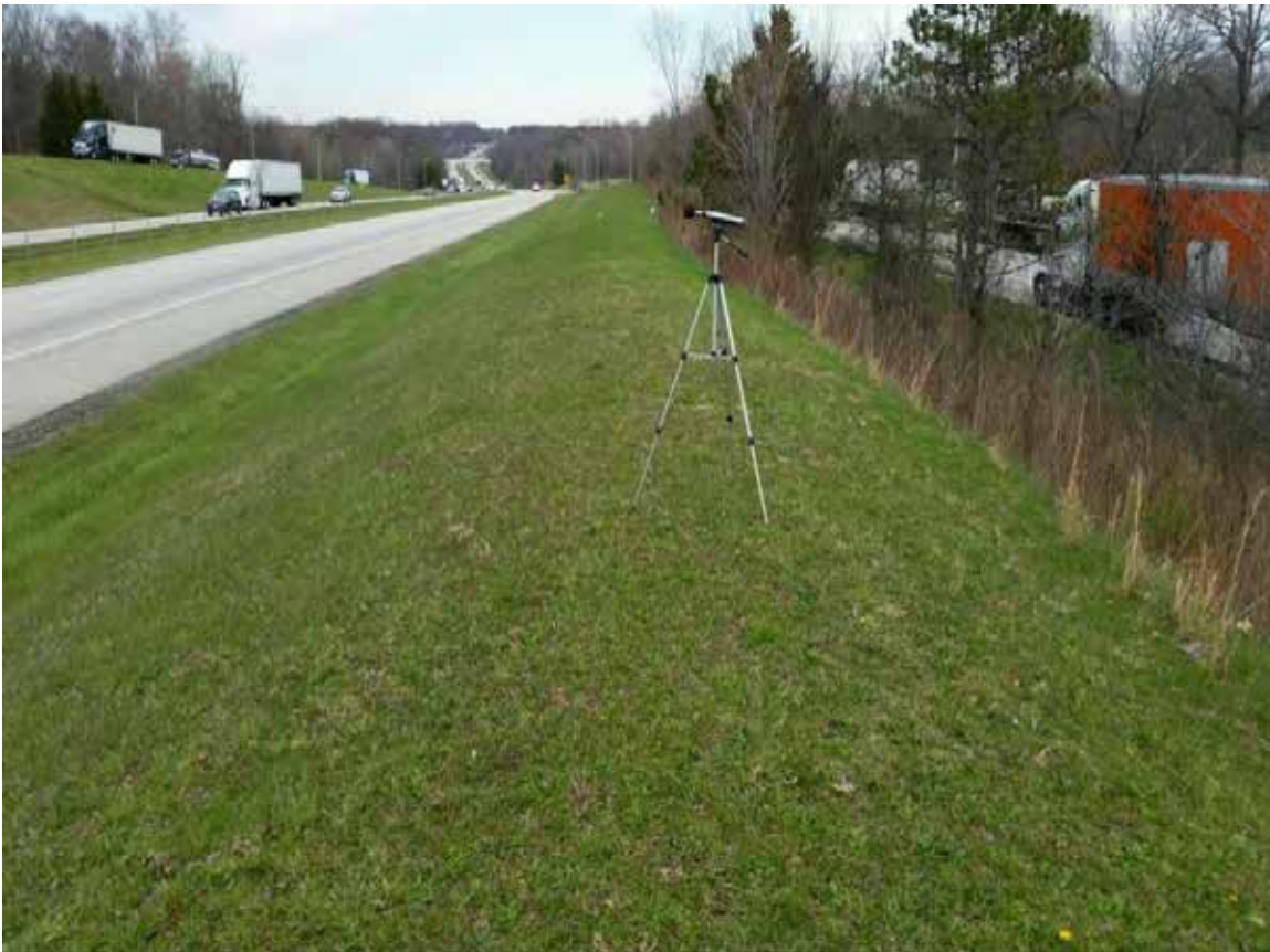
Site 12: POR-76 EB, Rest Area (between Porter and Alliance Roads), Looking along Noise Berm Northern Slope
