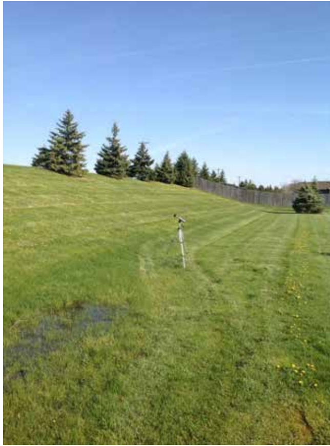
Site 13: MIA-75 NB, Foxtail Circle, Looking along Noise Berm Eastern Slope
