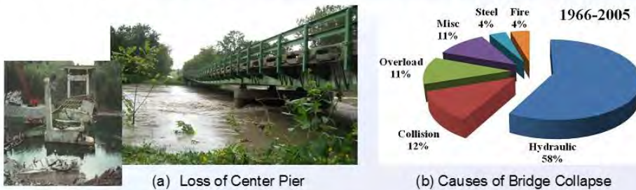
Fig. 10 Scour-Induced Bridge Damage and Statistics
