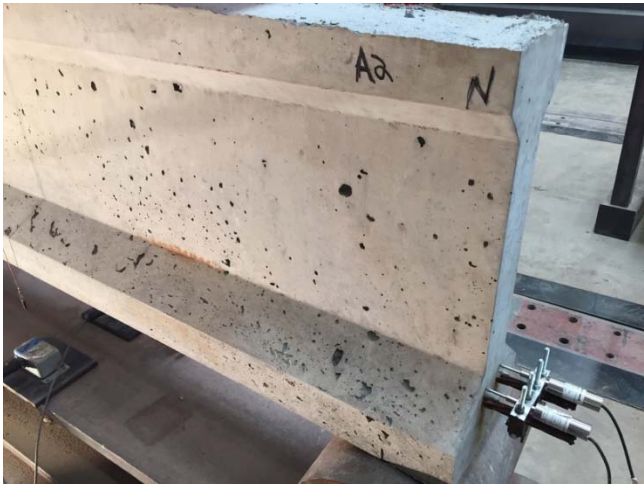
Figure 8-46: Condition of specimen A2N prior to testing
