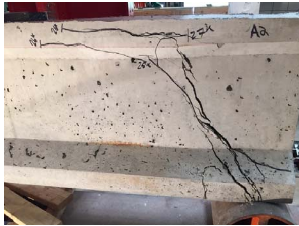
Figure 8-49: Cracking along the flange and web for specimen A2N
