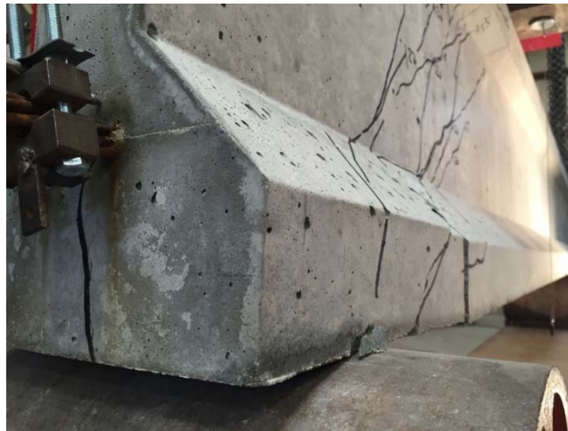
Figure 8-41: Cracking near the support and in the end of specimen C3S
