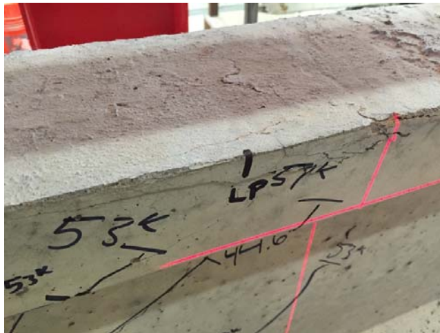
Figure 8-37: Concrete crushing at top of top flange at failure of specimen C3NC
