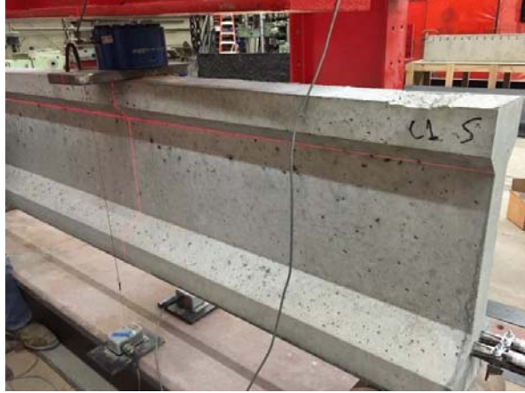
Figure 8-15: Specimen C1S before shear testing
