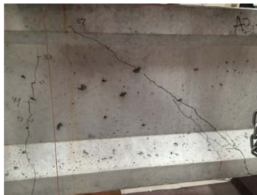
Figure 8-21: Visual map of cracking for shear test of specimen A3SC
