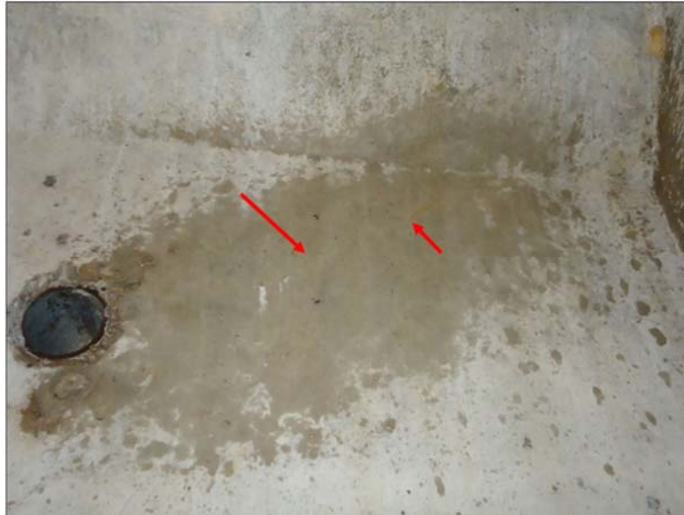
Figure D-18: Hairline diagonal cracks from top flange/web interface towards pipe on interior beam (5W-N)
