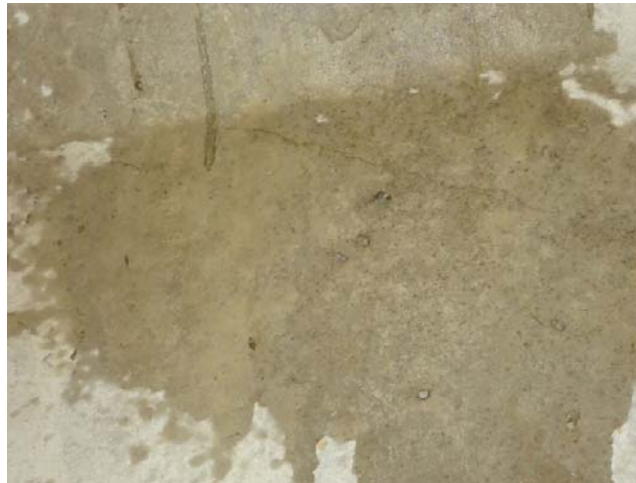
Figure D-69: Diagonal web crack extending from top flange and web intersection (5N-W)
