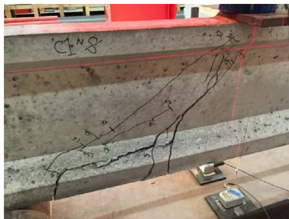
Figure 8-13: Visual map of cracking for shear test of specimen C1NC
