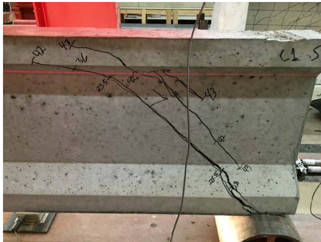
Figure 8-19: Visual map of cracking for shear test of specimen C1S
