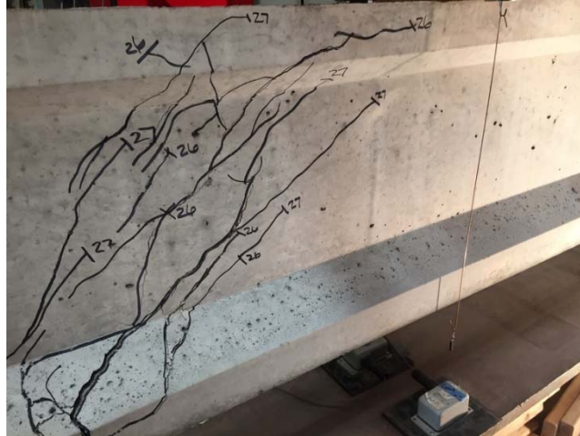
Figure 8-40: Visual map of cracking for specimen C3S
