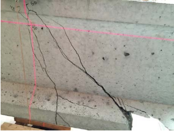
Figure 8-24: Visual map of cracking for shear test of specimen A3N
