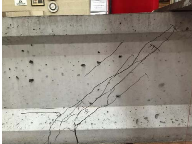
Figure 8-32: Visual map of cracking for shear test of specimen C2S
