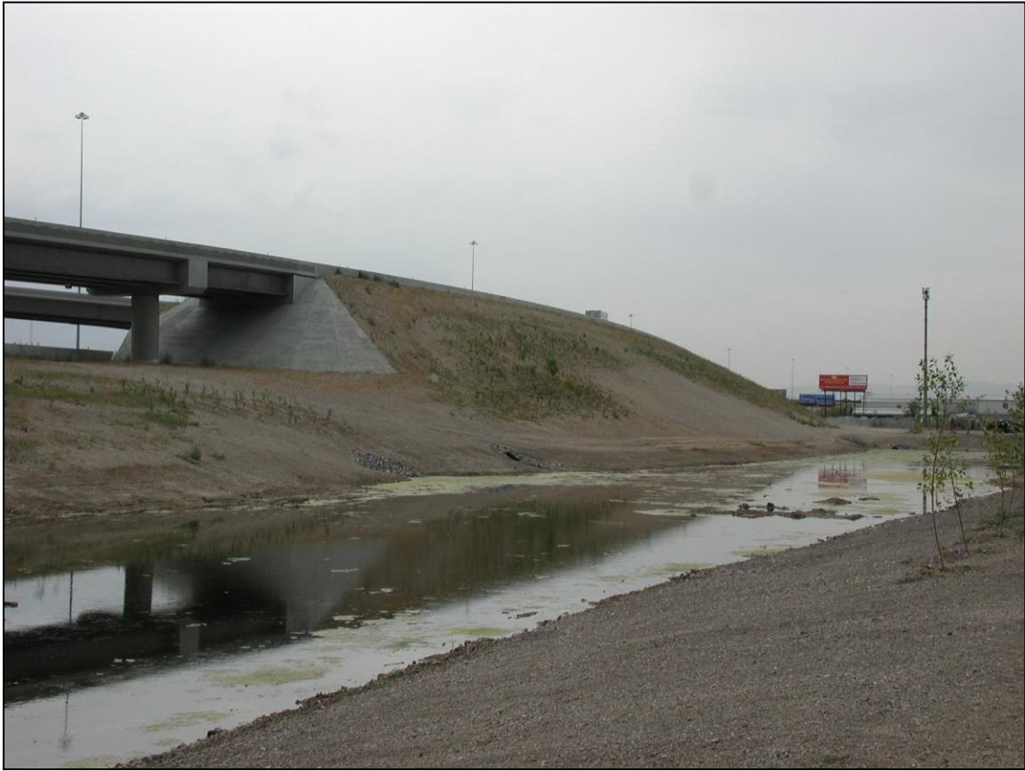
Figure 4-19. I-15 Merger large earth embankment.
