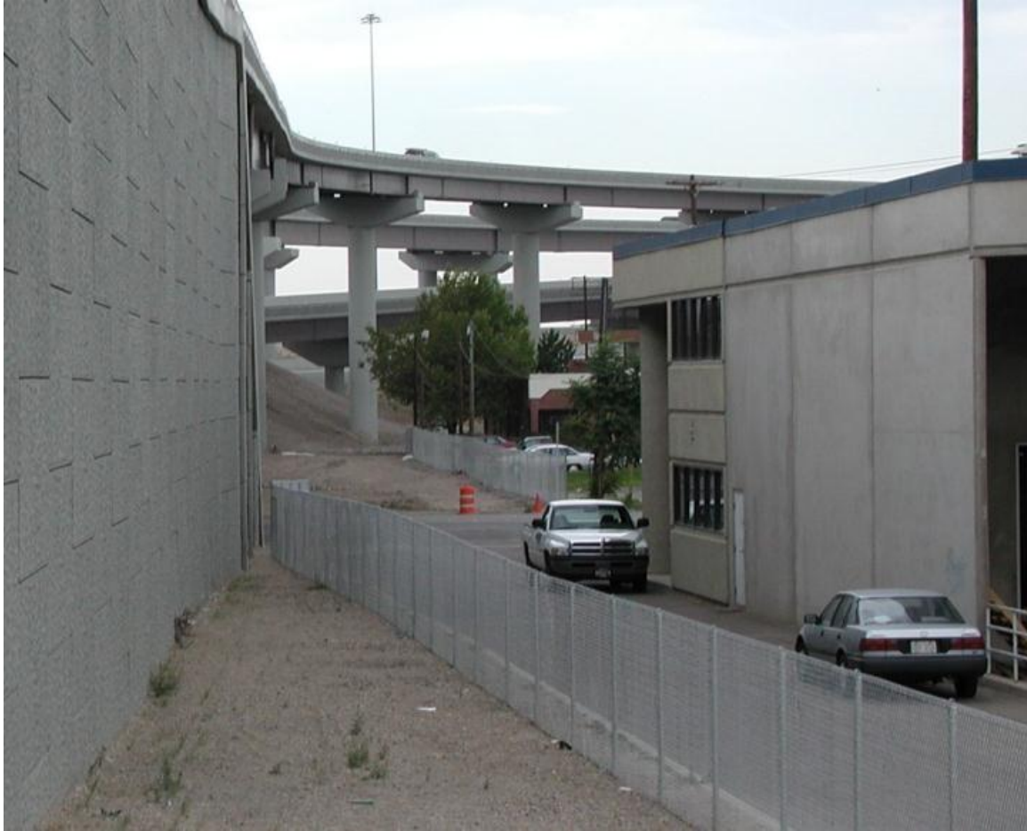
Figure 4-1. LCC stabilized foundation site and adjacent building.
