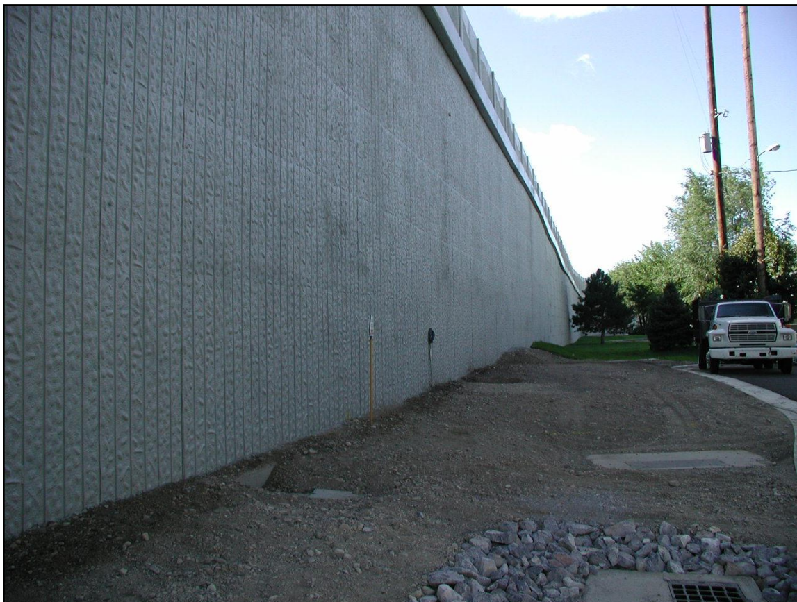
Figure 4-11. 100 South geofabric embankment.
