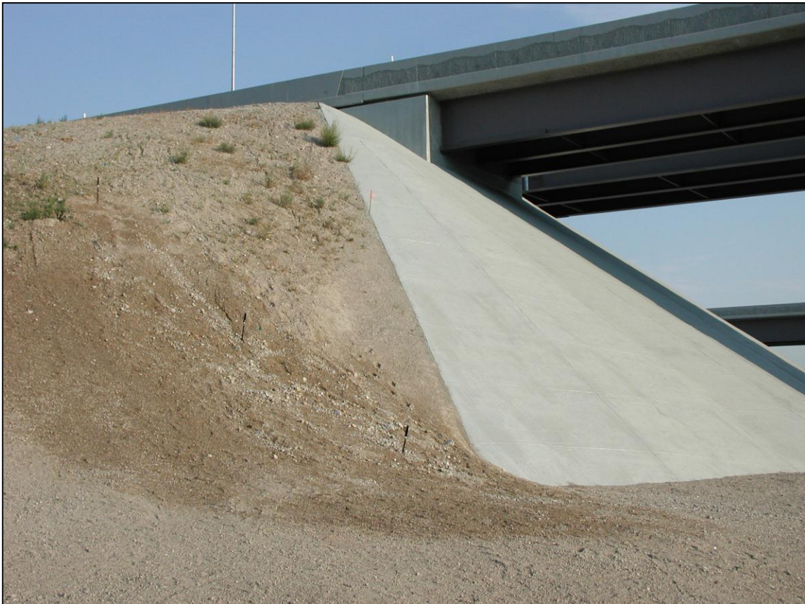
Figure 4-18. 900 West large earth embankment.
