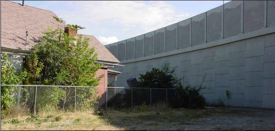
Figure 4-5. Proximity of residential structure adjacent to the 200 South MSE wall.
