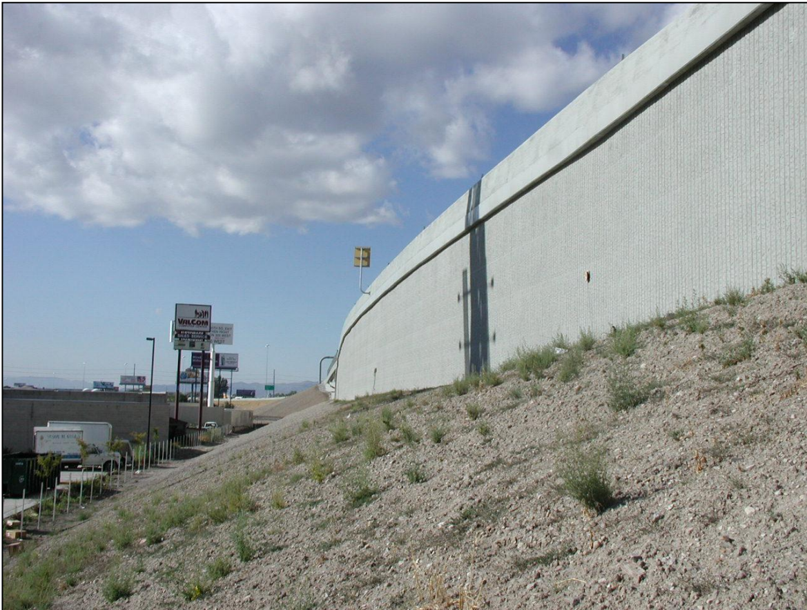
Figure 4-10. 3300 South geofabric embankment with toe berm.
