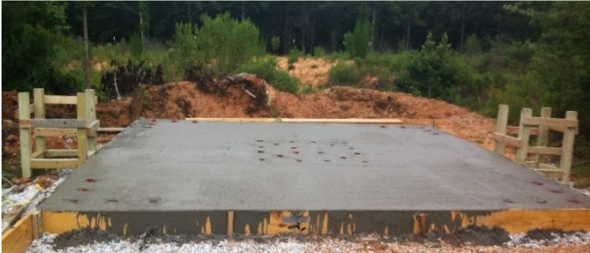
Figure 3-8: A Completed Slab
