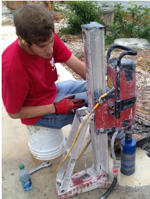
Figure 3-12: Drilling of a Core from the Exterior Region of a Slab
