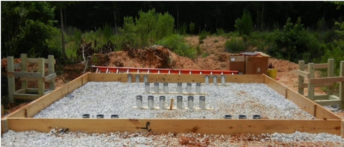
Figure 3-7: Typical Setup before Placement
