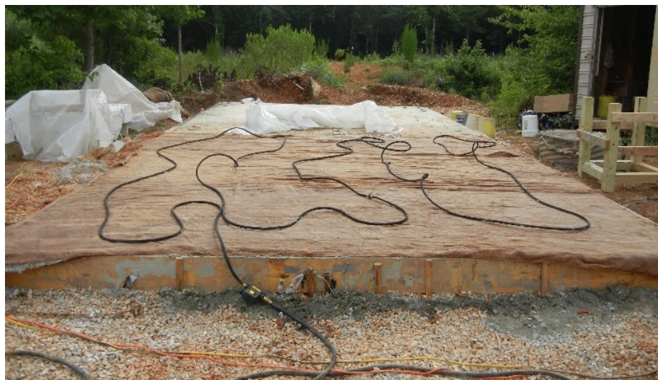
Figure 3-9: Curing Mats and Soaker Hoses
