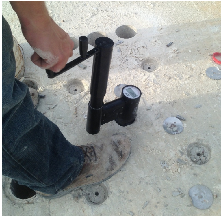
Figure 3-15: Pullout Test Being Performed
