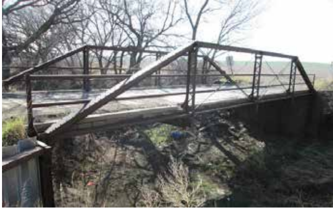
Figure 5.38: Old Steel-Truss Bridge, Which was Closed in June 2015
