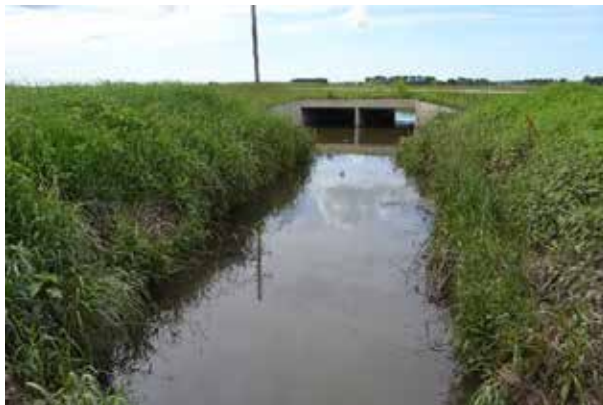
Figure 5.43: View of Structure from Downstream
