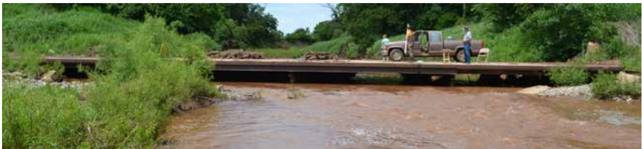
Figure 5.62: View of Bridge from Downstream
