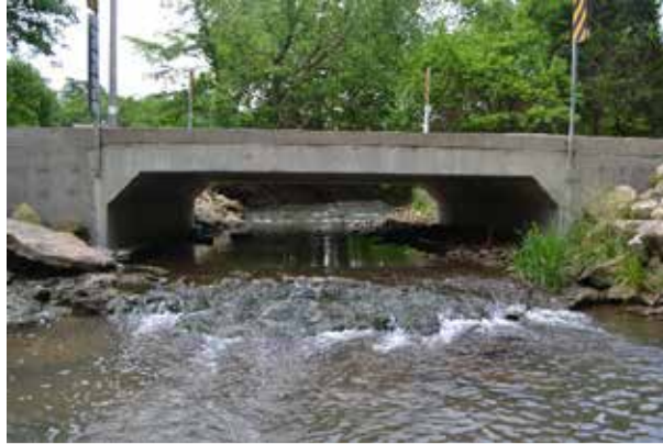
Figure 5.50: View of Structure from Downstream
