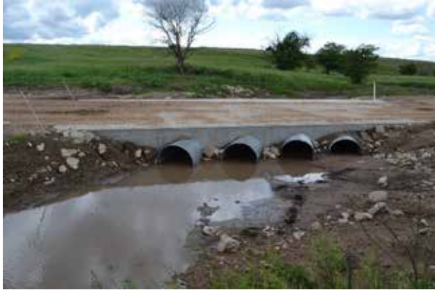
Figure 5.19: View of Structure from Downstream
