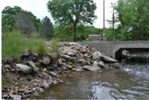
Figure 5.56: Downstream Face and East Abutment
