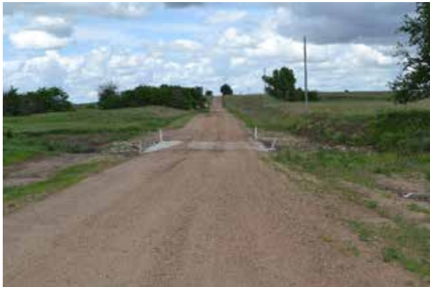
Figure 5.20: View of Crossing from Road
