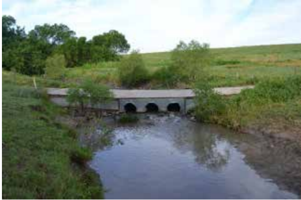
Figure 5.30: View of Structure from Downstream
