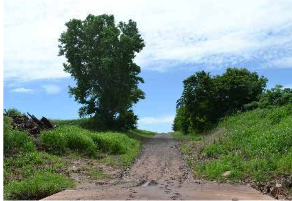
Figure 5.69: South Approach Viewed from Bridge
