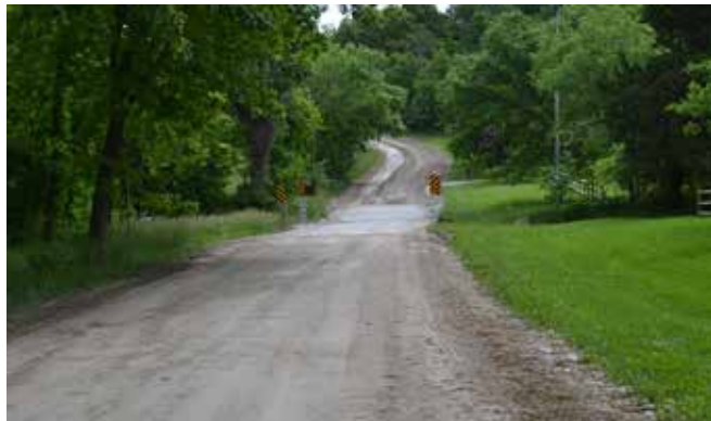
Figure 5.51: View of Crossing from 175th
