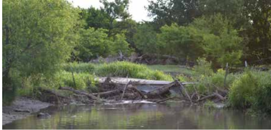
Figure 2.1: Woody Debris Trapped on Upstream Side of Vented Ford in Phillips County, Kansas
