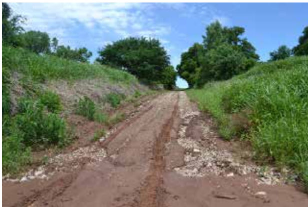
Figure 5.68: North Approach Viewed from Bridge
