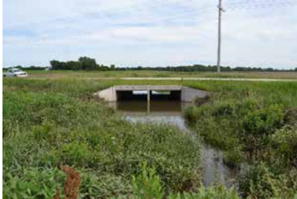
Figure 5.42: View of Structure from Upstream
