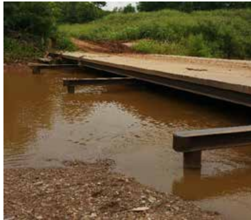
Figure 5.70: Debris-Trapping Piers on the Upstream Side of Bridge
