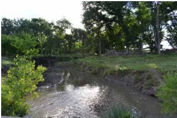
Figure 5.32: Downstream Channel Viewed from Deck of Structure
