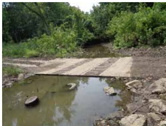
Figure 5.9: View of Structure from Upstream
