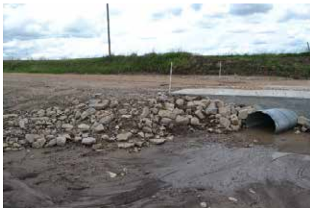
Figure 5.24: Bank Stabilization and Silt Accumulation on Downstream Side of Structure
