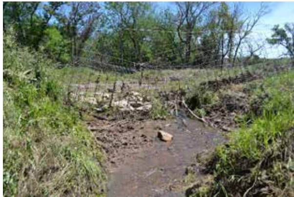
Figure 5.3: View of Structure from Downstream
