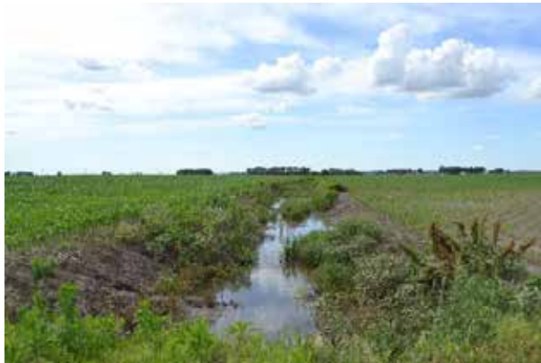
Figure 5.46: Channel Directly Upstream of the Culvert
