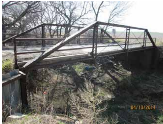
Figure 1.1: Recently Closed Steel Truss Bridge in Osborne County, Kansas
