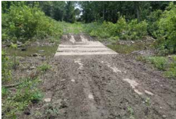
Figure 5.11: View of Structure Looking South
