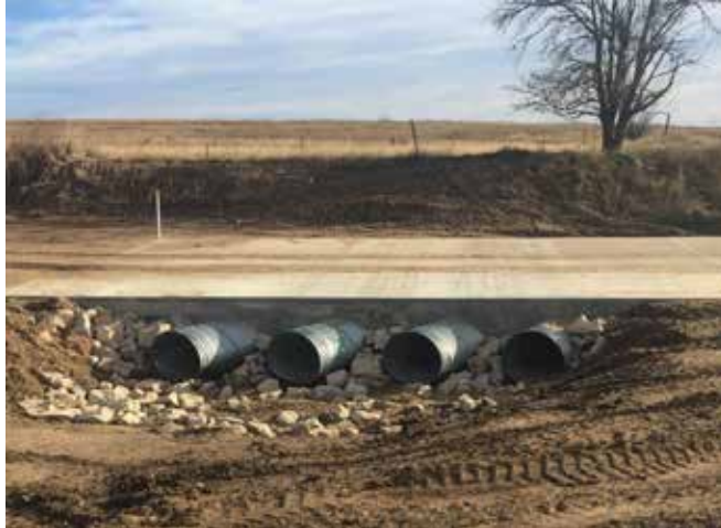
Figure 1.3: Vented Ford in Kiowa County, Kansas
