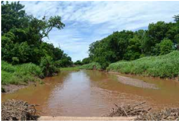
Figure 5.64: View of Upstream Channel from Bridge
