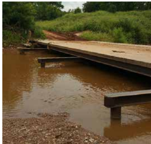
Figure 1.7: Low-Profile Open-Span Bridge in Sumner County, Kansas
