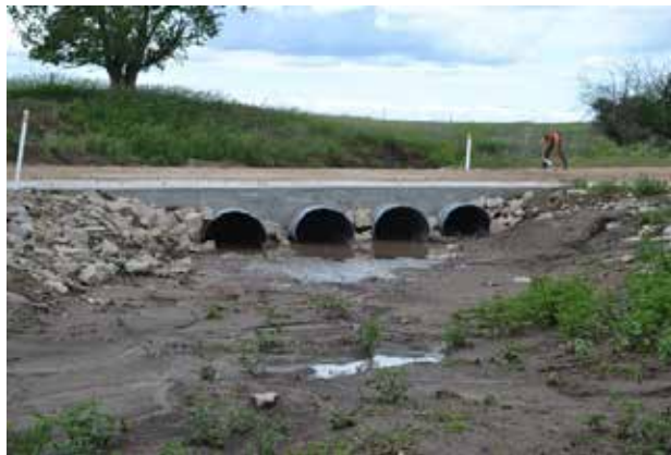
Figure 5.18: View of Structure from Upstream
