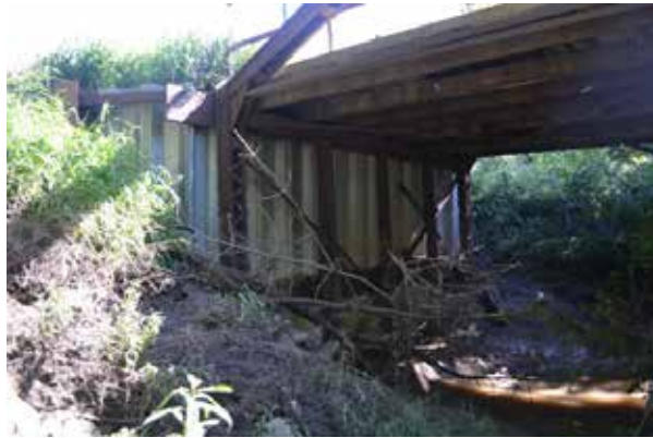
Figure 5.39: Left Abutment Retrofitted with Steel Sheet-Pile
