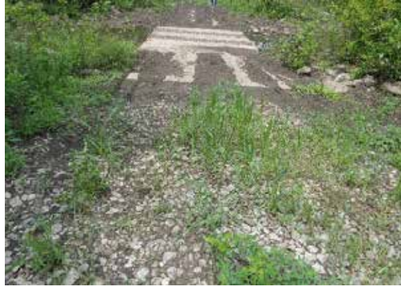
Figure 5.16: Rock Surface Material on South Approach
