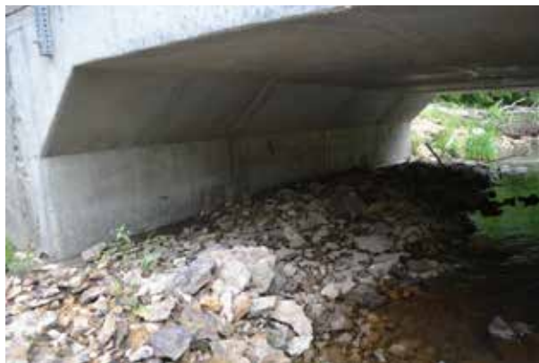
Figure 5.52: West Abutment from Downstream Side
