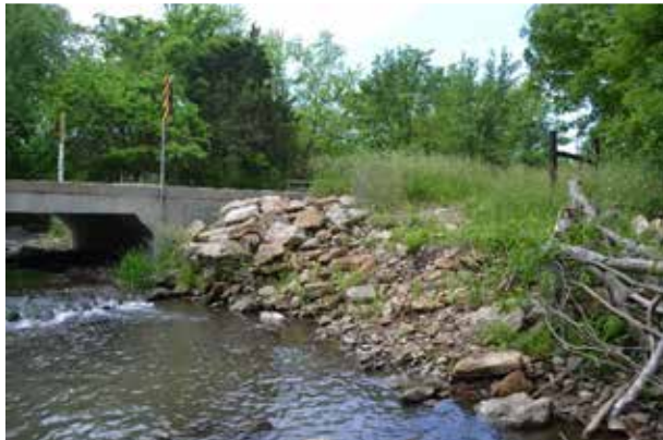
Figure 5.57: Downstream Face and West Abutment
