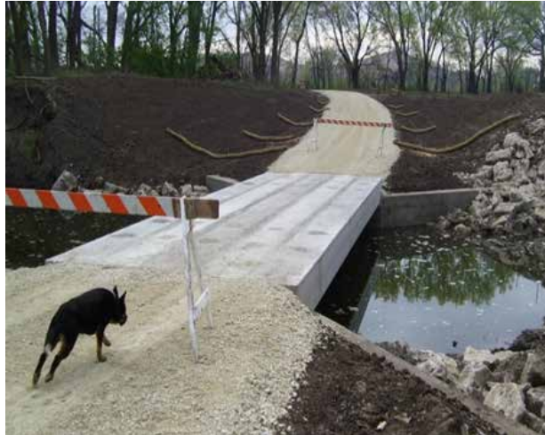
Figure 1.6: Low-Profile Open-Span Bridge in Geary County, Kansas
