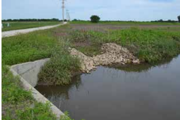
Figure 5.45: Downstream Wingwall with Riprap Stabilization
