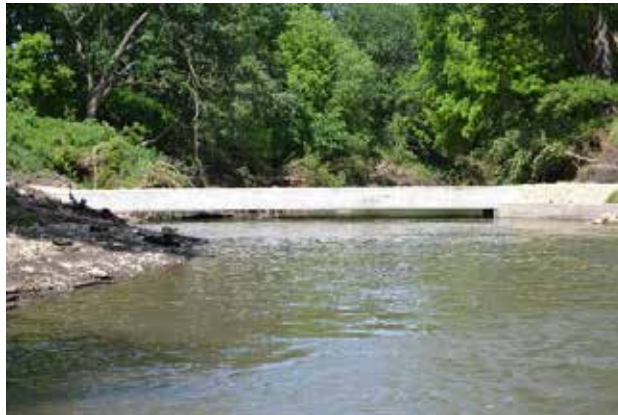
Figure 5.75: View of Structure from Upstream
