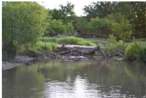
Figure 5.29: View of Structure from Upstream
