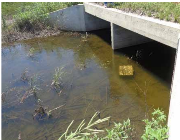
Figure 1.4: Low-Profile Box Culvert in Shawnee County, Kansas
