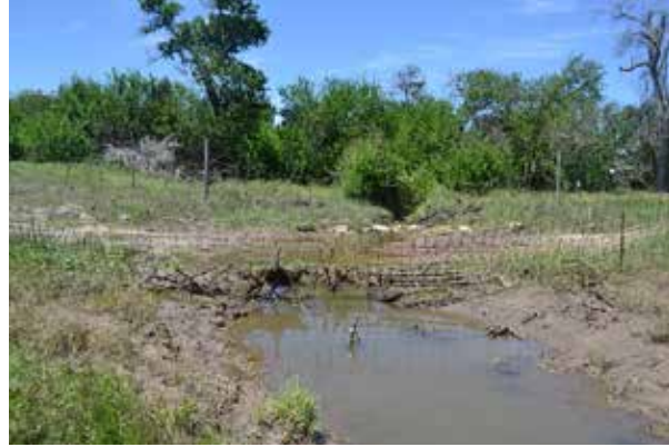
Figure 5.2: View of Structure from Upstream
