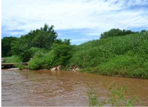
Figure 5.66: View of Downstream Bridge Face in Comparison to Streambank Height
