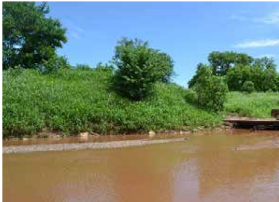
Figure 5.67: View of Upstream Bridge Face in Comparison to Streambank Height
