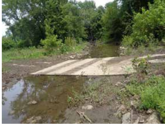
Figure 5.10: View of Structure from Downstream
