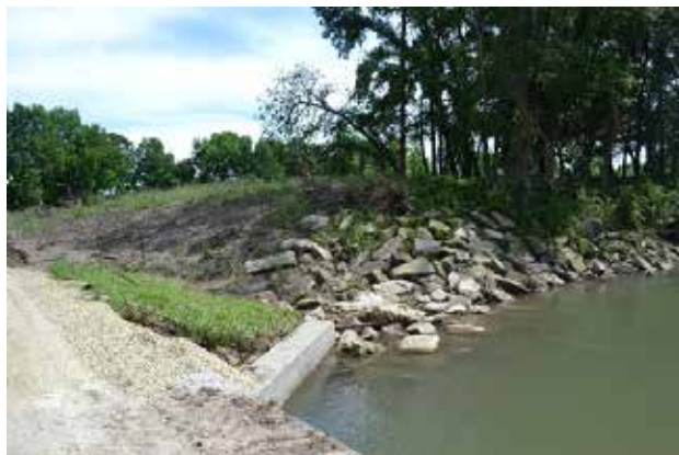
Figure 5.78: Upstream Right Bank
