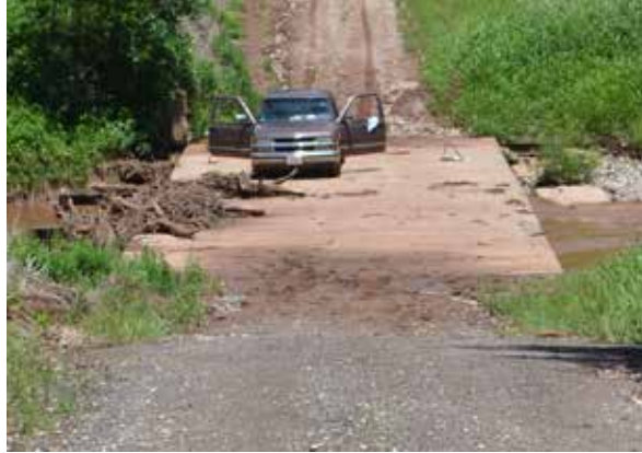
Figure 5.63: View of Bridge from Road
