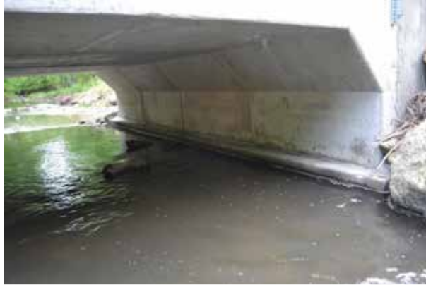
Figure 5.53: East Abutment from Downstream Side, Showing Exposure of Stem Wall
