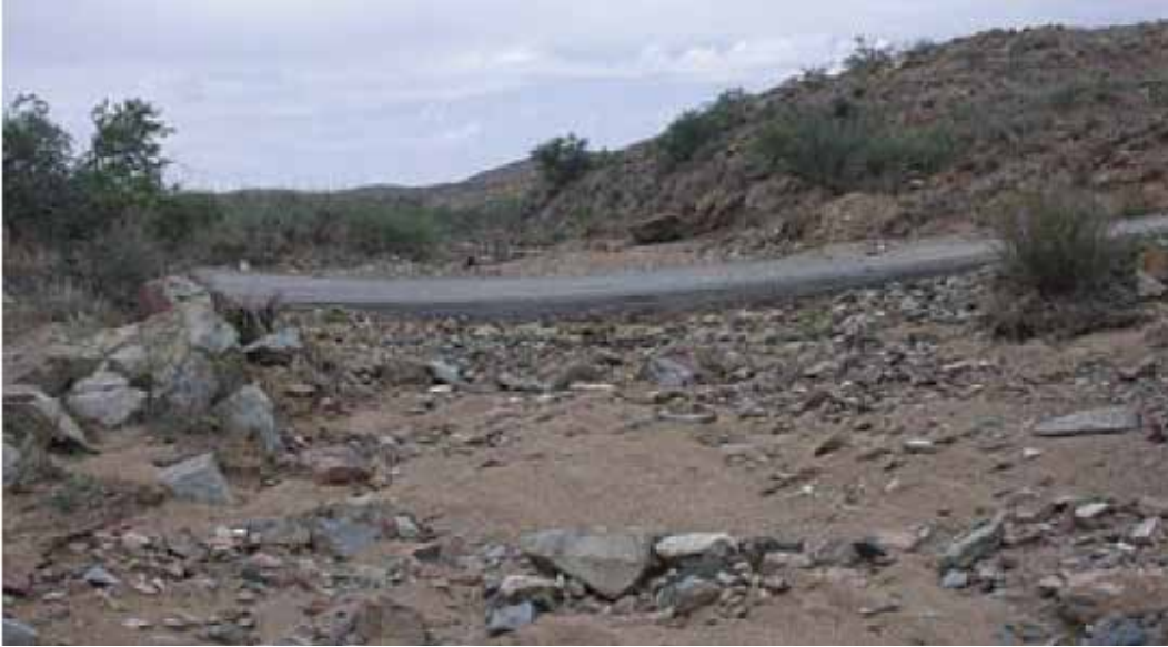
Figure 1.2: Unvented Ford on an Ephemeral Tributary of the Agua Fria River in Arizona Source: Clarkin et al. (2006)
