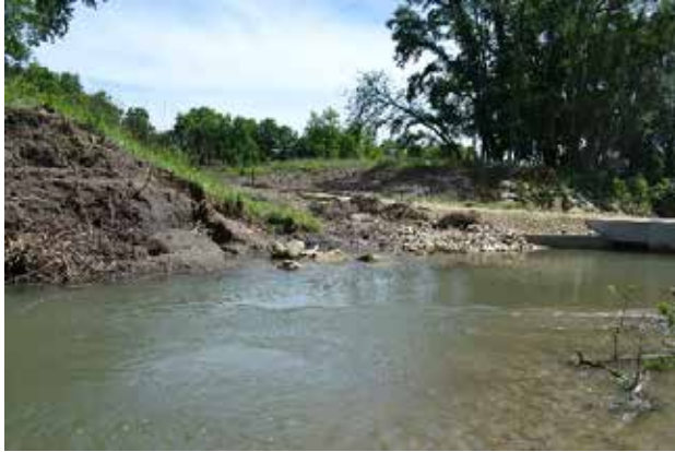
Figure 5.85: Right Bank Downstream of Bridge, Looking Toward Bridge
