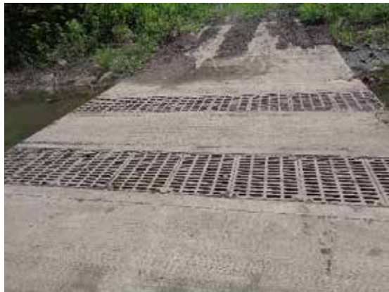
Figure 5.15: Close-Up View of the Grated Troughs
