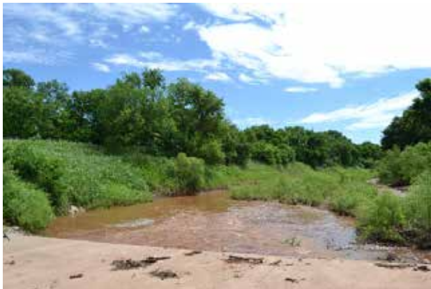
Figure 5.65: View of Downstream Channel from Bridge
