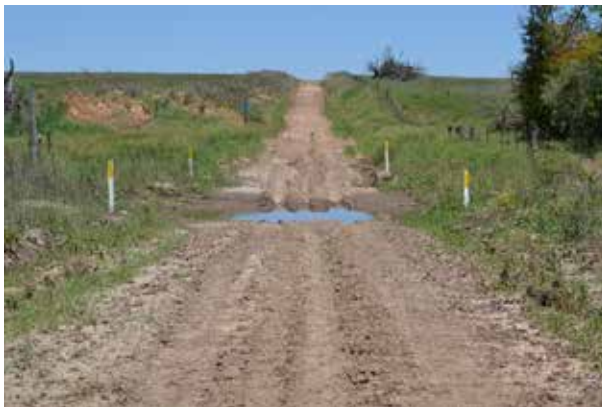
Figure 5.4: View of Structure from Road
