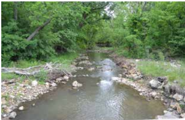
Figure 5.55: Downstream Channel Viewed from Structure
