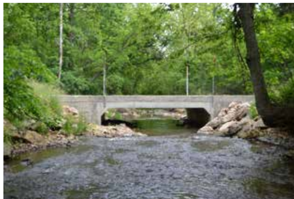
Figure 5.49: View of Structure from Upstream
