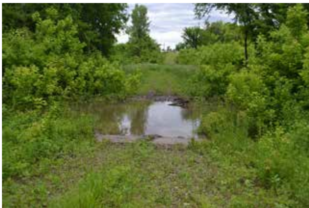
Figure 5.12: View of Submerged Structure Looking North
