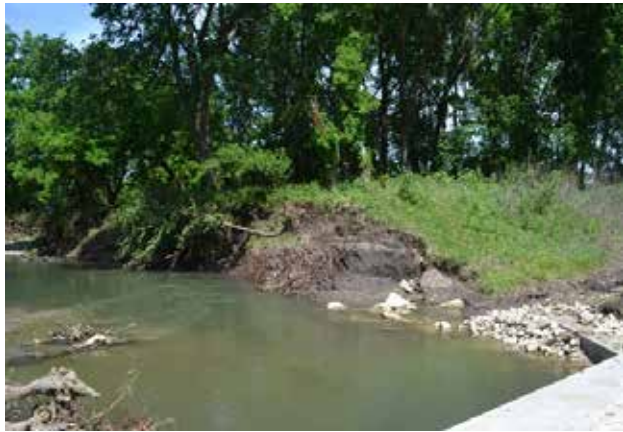
Figure 5.80: Downstream Right Bank
