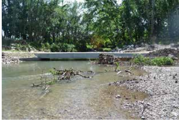
Figure 5.76: View of Structure from Downstream
