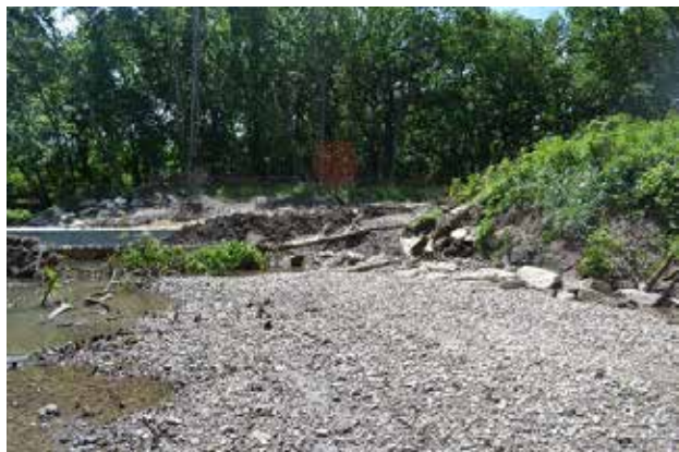
Figure 5.84: Left Bank Downstream of Bridge, Looking Toward Bridge
