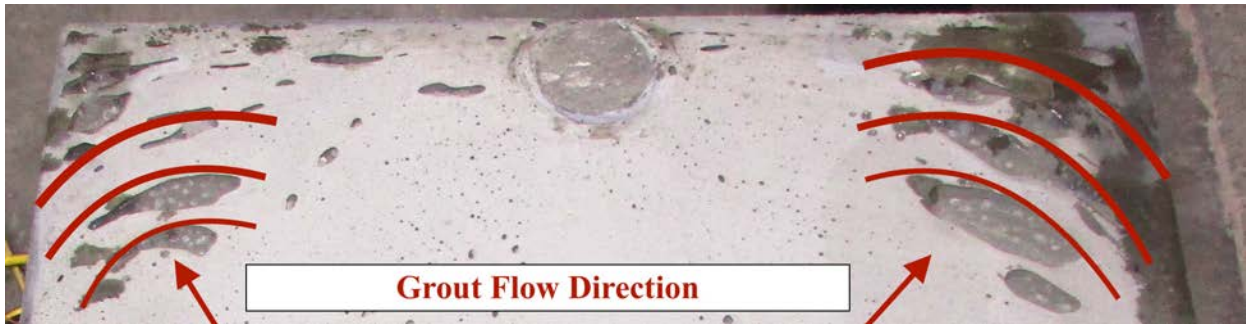
Figure 4.14: Air void pattern indicate the grout flow (for mockup specimen MU3)
