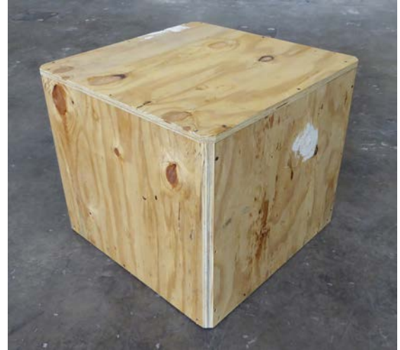
(b) Inner formwork — pile head
