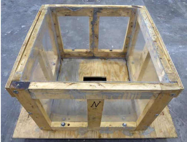
(a) Outer formwork — bent cap pile-pocket
