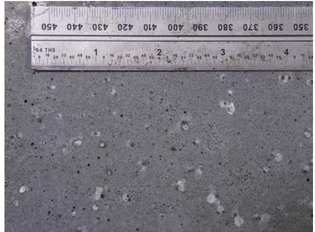
(b) Detail — Closeup of North West
