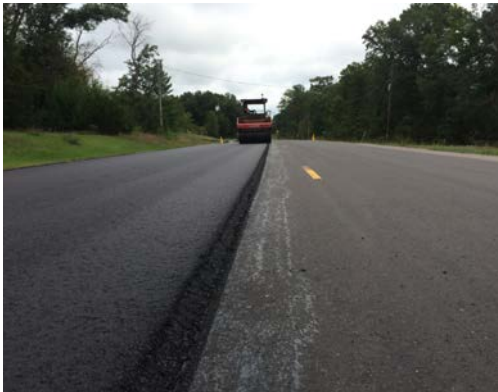
(b) rolling unconfined joint
