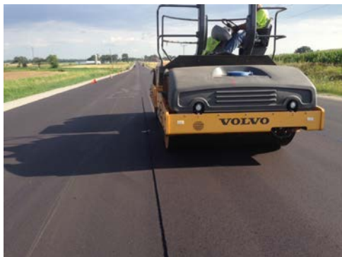
(b) 12-inches away, pass 1, section 2 Figure 34 STH 26 confined edge
