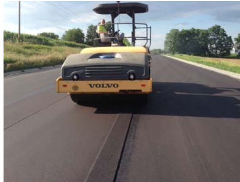
(c) 3-inch overlap, pass 2, section 2
