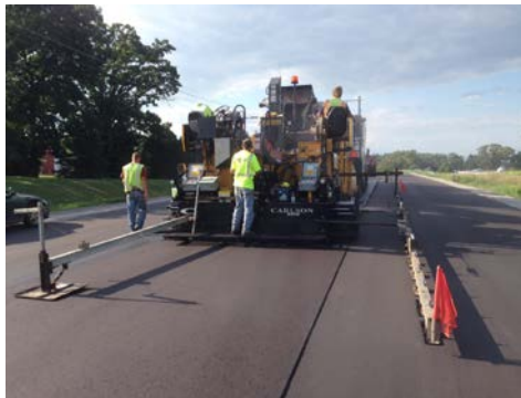
(a) STH 26 confined joint
