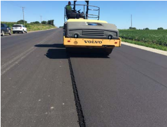
(c) 3-inch overhang, pass 2, section 1
