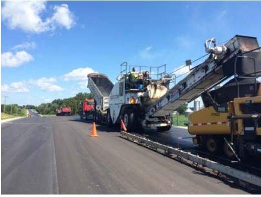
(a) STH 26 paving train using a ski
