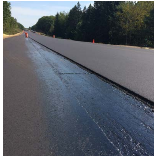
(b) Sufficient tack
