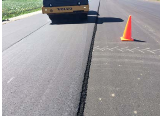
(b) Test section divider (facing north)
